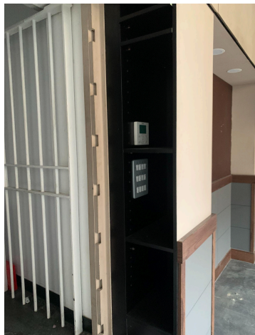
11 - non original column and wall lining to be removed -vault gate to be retained
