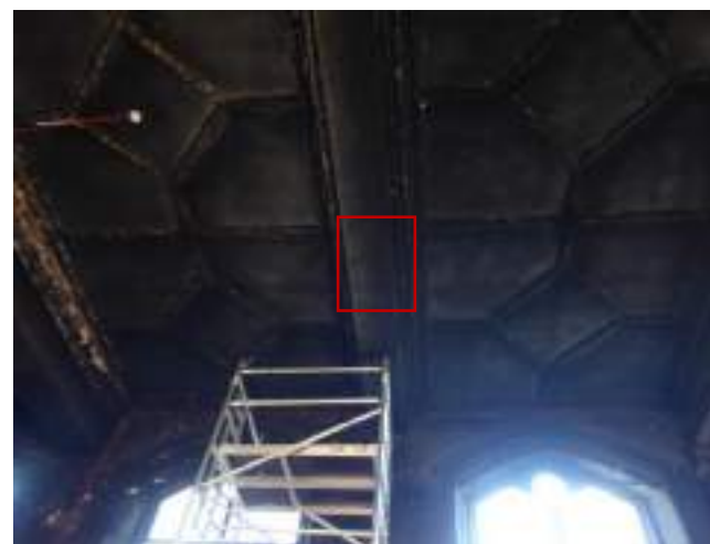
Figure 18: section of ceiling showing suspected area of additional plaster skim.
