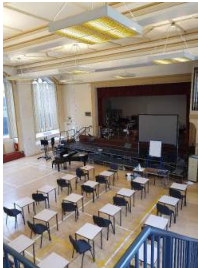
Figure 12: Whiteley Hall prior to fire damage (supplied by the school)
