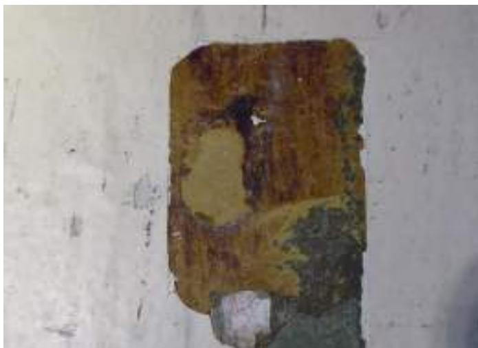
Figure 27: image of exposed yellow scheme with darkened coating applied over.
