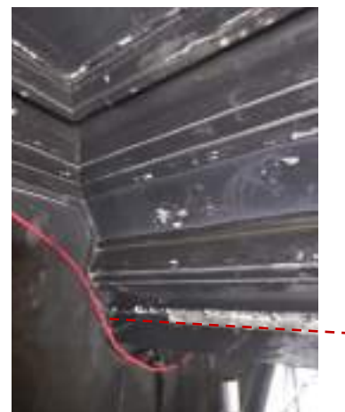
Figure 18: section of ceiling showing suspected area of additional plaster skim.
