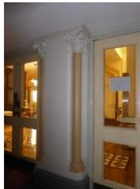
Figure 21: image of the entrance vestibule to the main entrance foyer as seen on the day of sampling.
