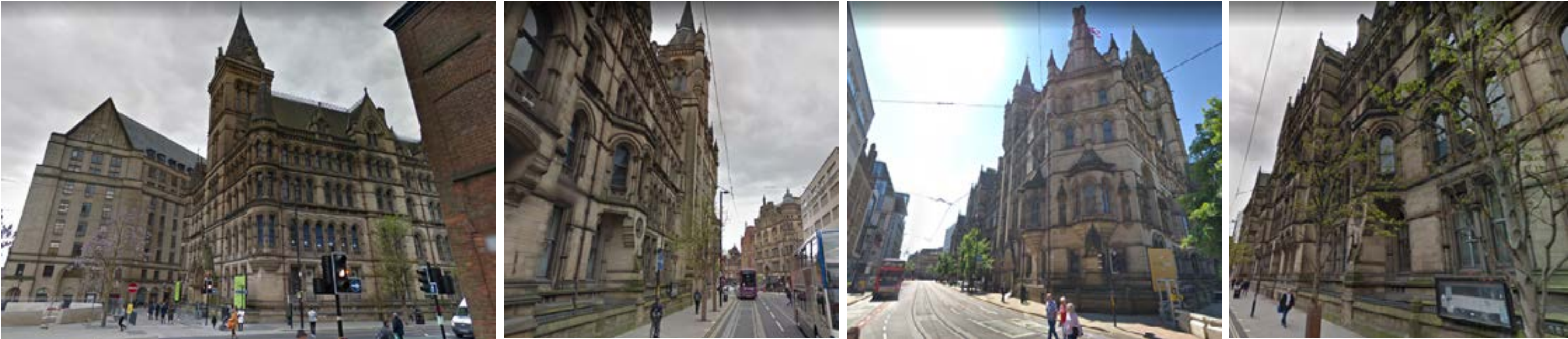
Princess Street Facade Obstructed view
