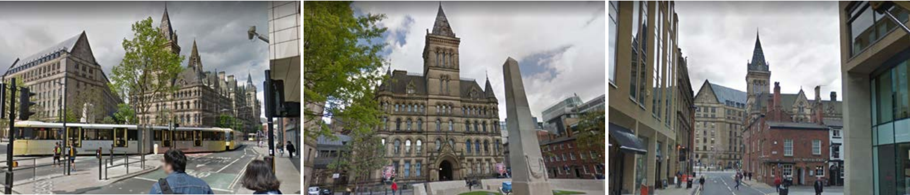
Cooper Street Facade Unobstructed view
