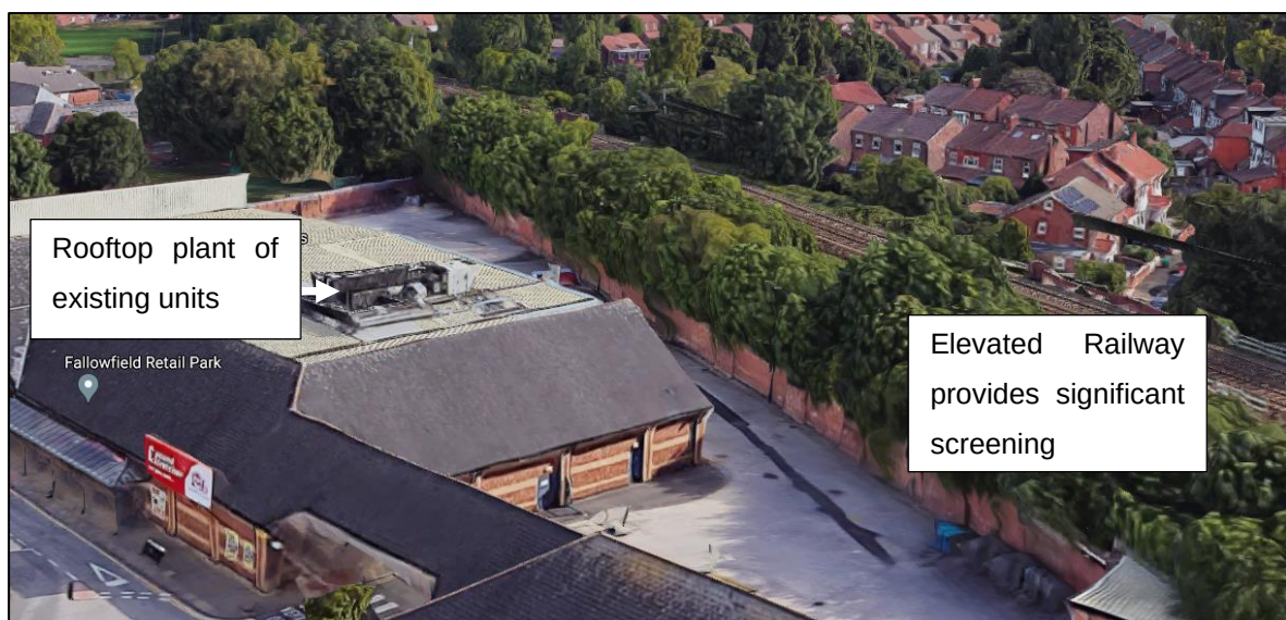
Figure 1: The existing site
