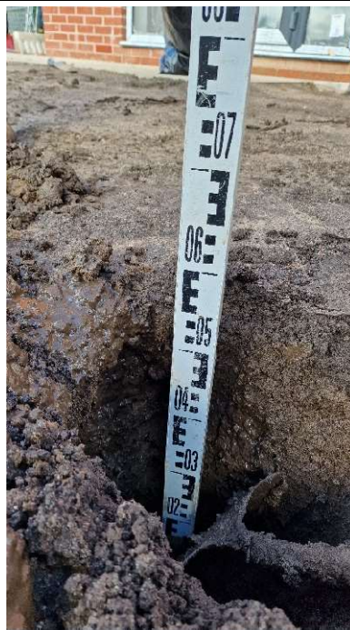
Close view of Staff - Total 600mm depth achieved.
