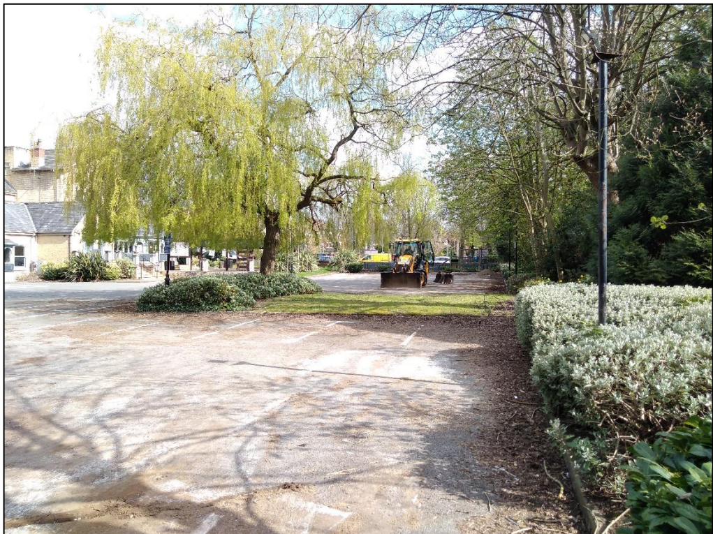
Photograph 02: Southwest corner of site looking east. April 2021
