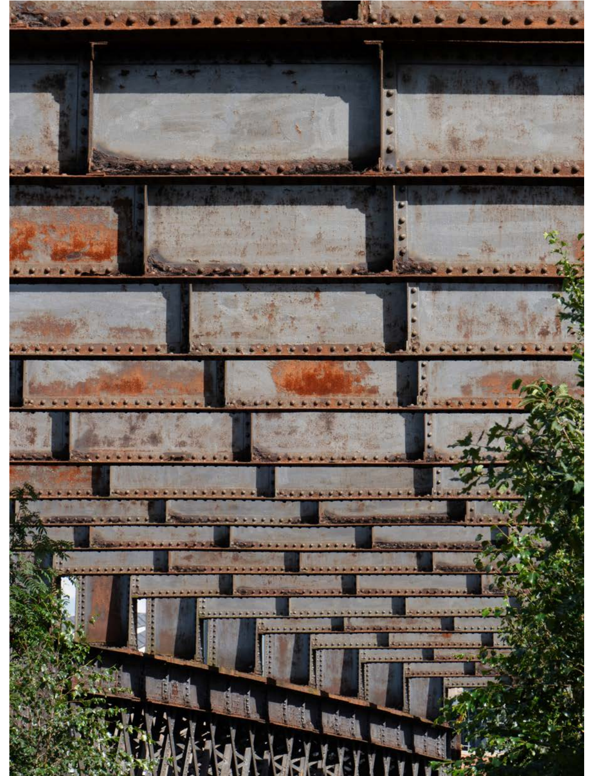
Castlefield Viaduct existing structure
