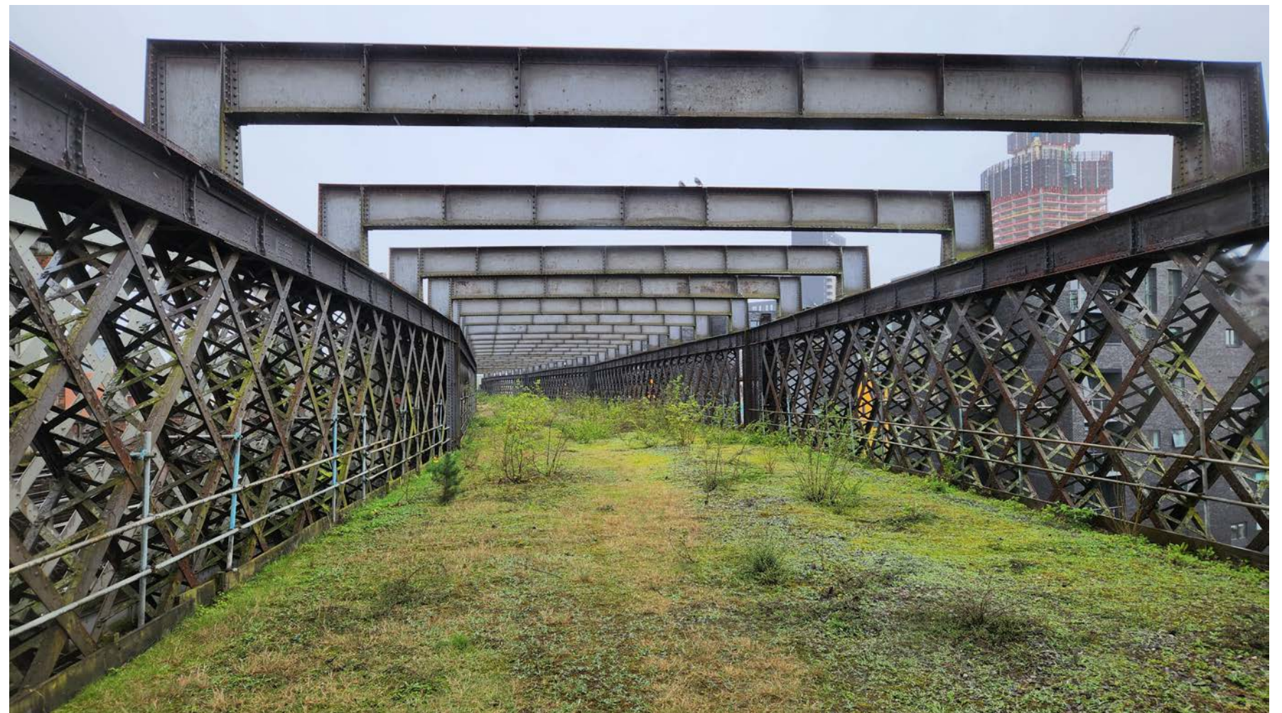
Original condition of Castlefield Viaduct
