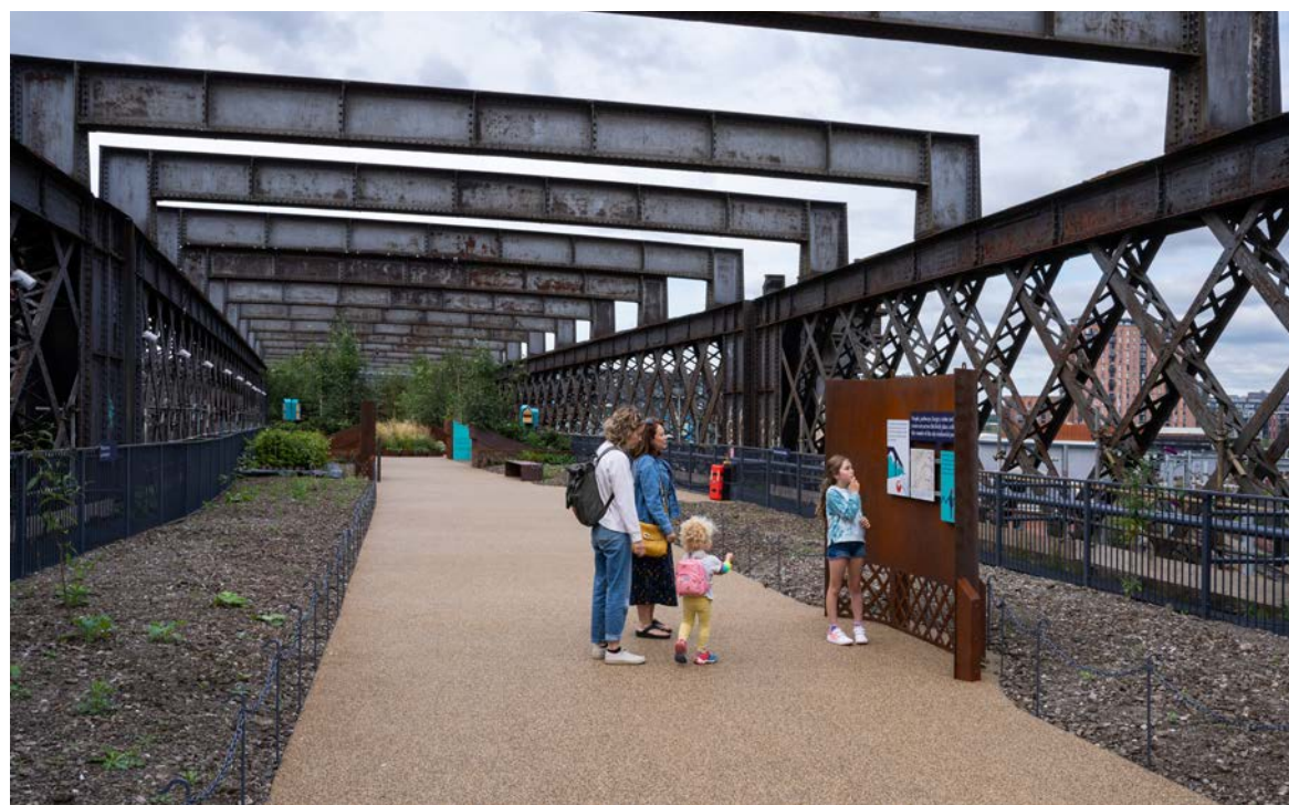
Phase 01 Naked Viaduct
