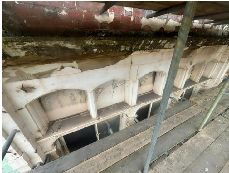
Example no. 5 – photo above showing upper second floor arched windows
