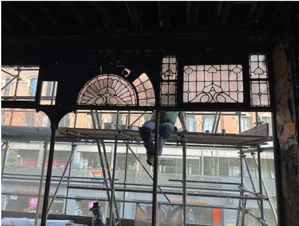
WIP example no. 1 above – cleaning and revealing of original first floor leaded windows
