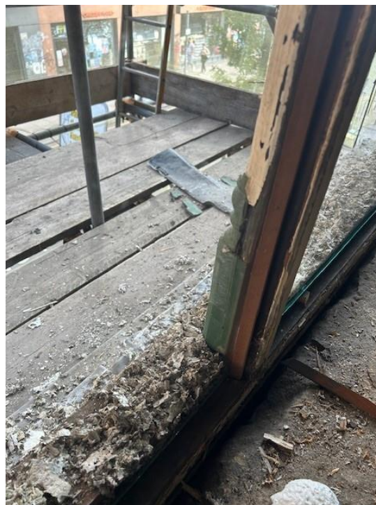
WIP example no. 2 above – combination of epoxy and slice repairs to rotten timber window frame mullions
