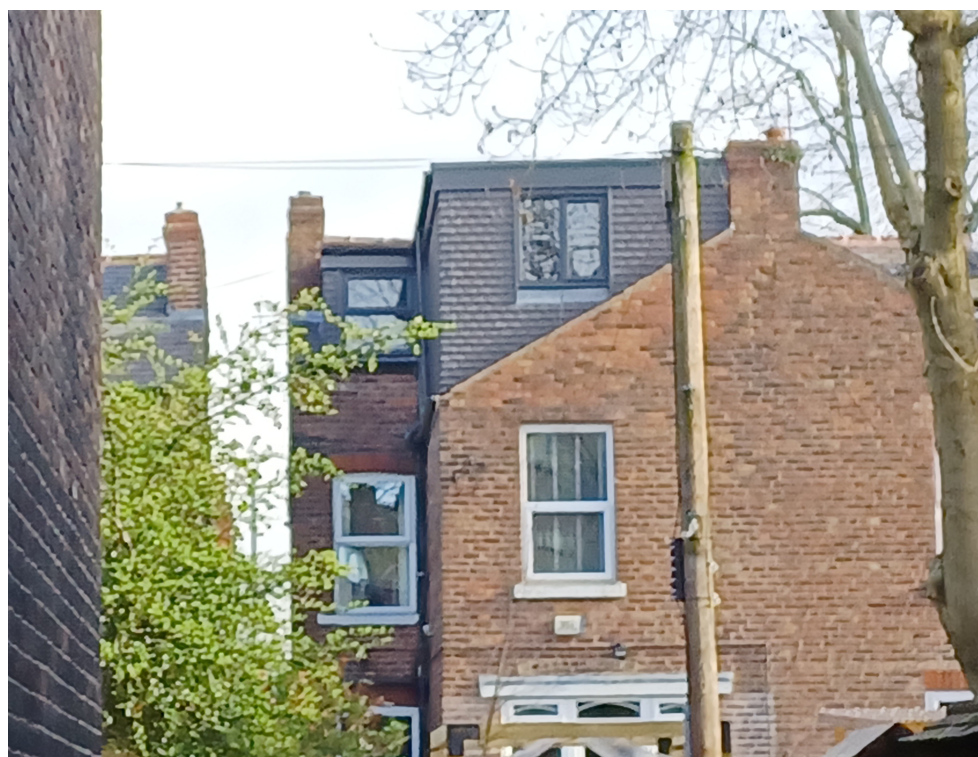
Figure 1. View of dormer in situ.
