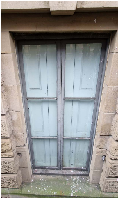
Typical External Photograph
