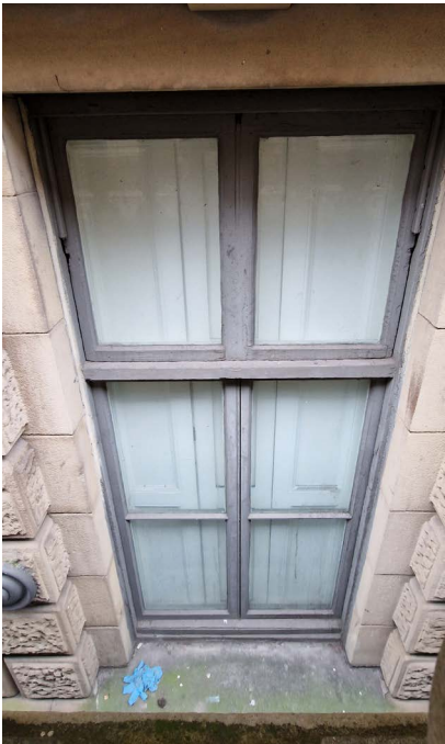
Typical External Photograph
