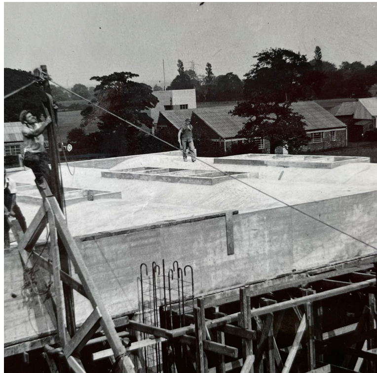
Image: Photograph of the roof at the rear of the Bus Garage, during original construction. From Manchester Bus Museum Archive.
