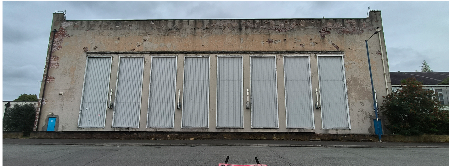
Image: External elevation to Harling Road
