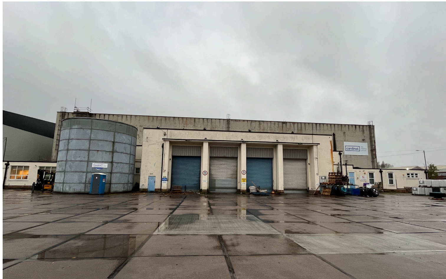
Image: Photograph of site, North East elevation.
