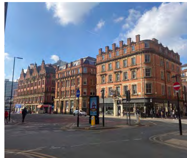
1.16 Corner of Port Street and Dale Street
