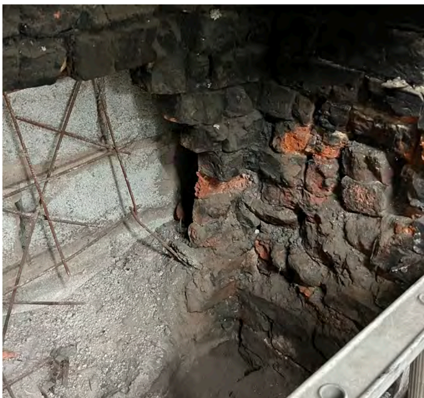
Fig 11. View inside rear Fireplace
