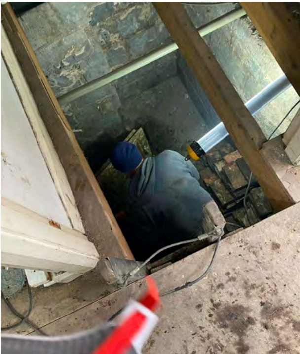
Fig.1 Opening in Ground floor, floor boards lifted to remove material from rear storeroom in basement. Breeze block walls and concrete visible.
