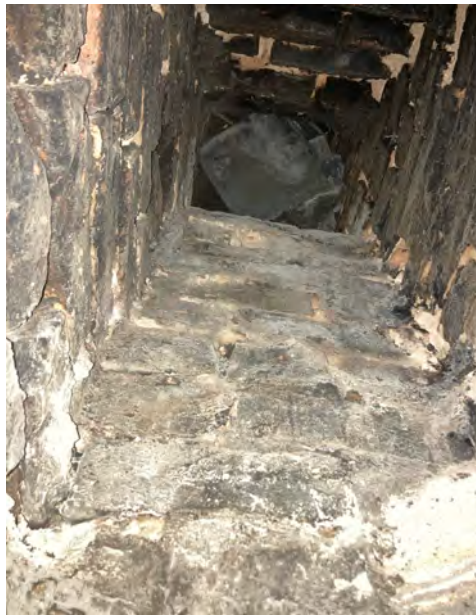
Fig 32. Removal of bricks exposed slates placed at the top.
