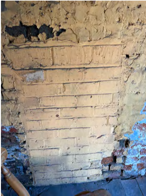
Fig 25. Rear Fireplace behind Painted brickwork.
