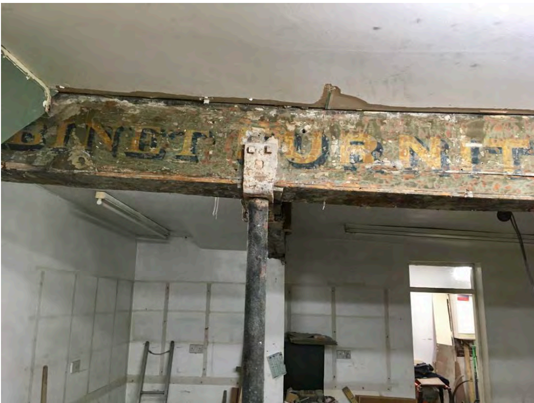
Fig 16. Original signage of suspected recycled beam. 'Cabinet furniture warehouse' Bracket covering part of original lettering.
