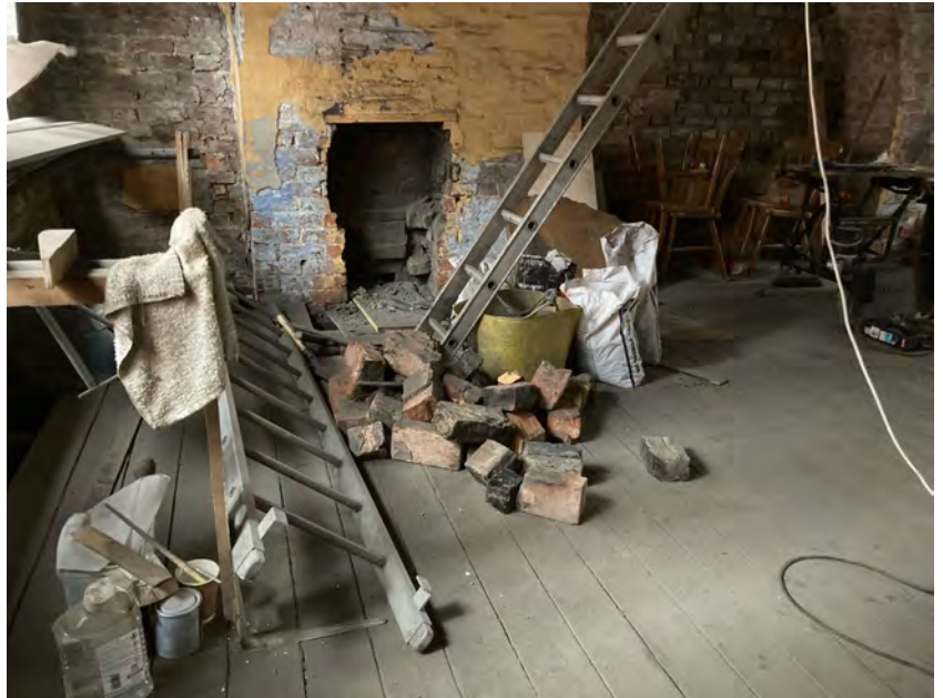
Fig 26. opening up of rear Fireplace
