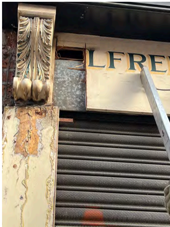
Fig 18. Behind the signage the metal housing of the roller shutter was revealed.
