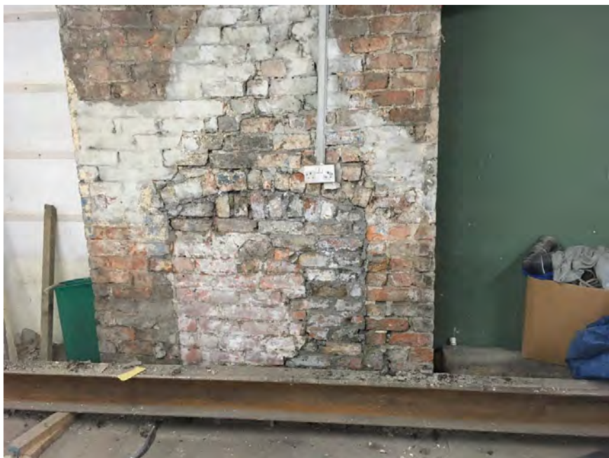
Fig 9. Rear Fireplace modern plaster removed.
