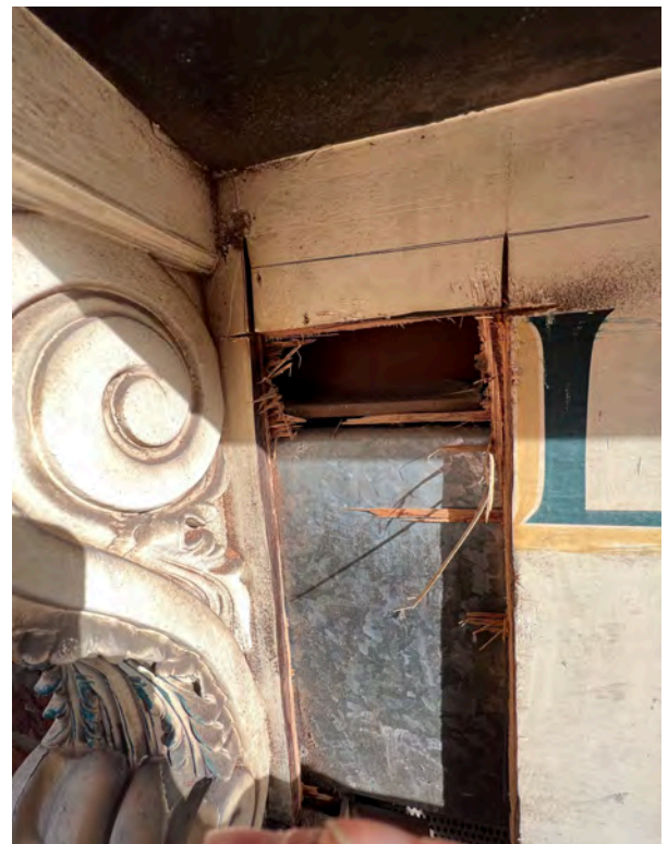
Fig 19. Above the metal roller shutter is a steel lintel, unfortunately no original signage found.
