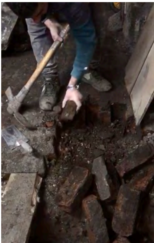
Fig 9. Bricks lifted by hand.
