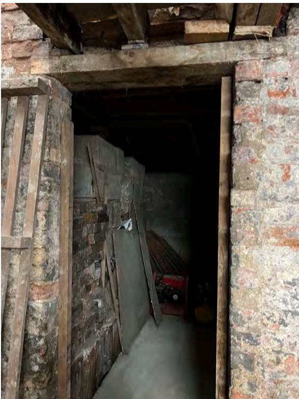
Fig.3 View into cleared rear store room. Salvaged bricks stacked on left side.
