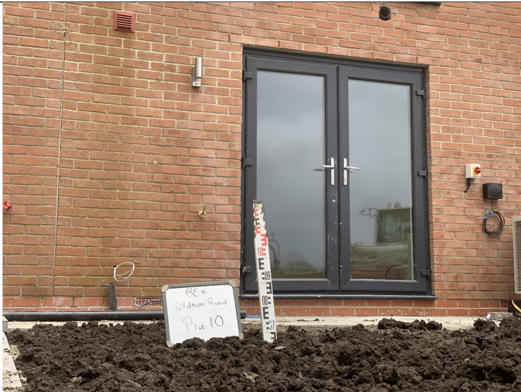
Photograph 2: Validation of Garden Capping
