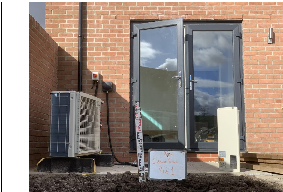
Photograph 2: Validation of Garden Capping
