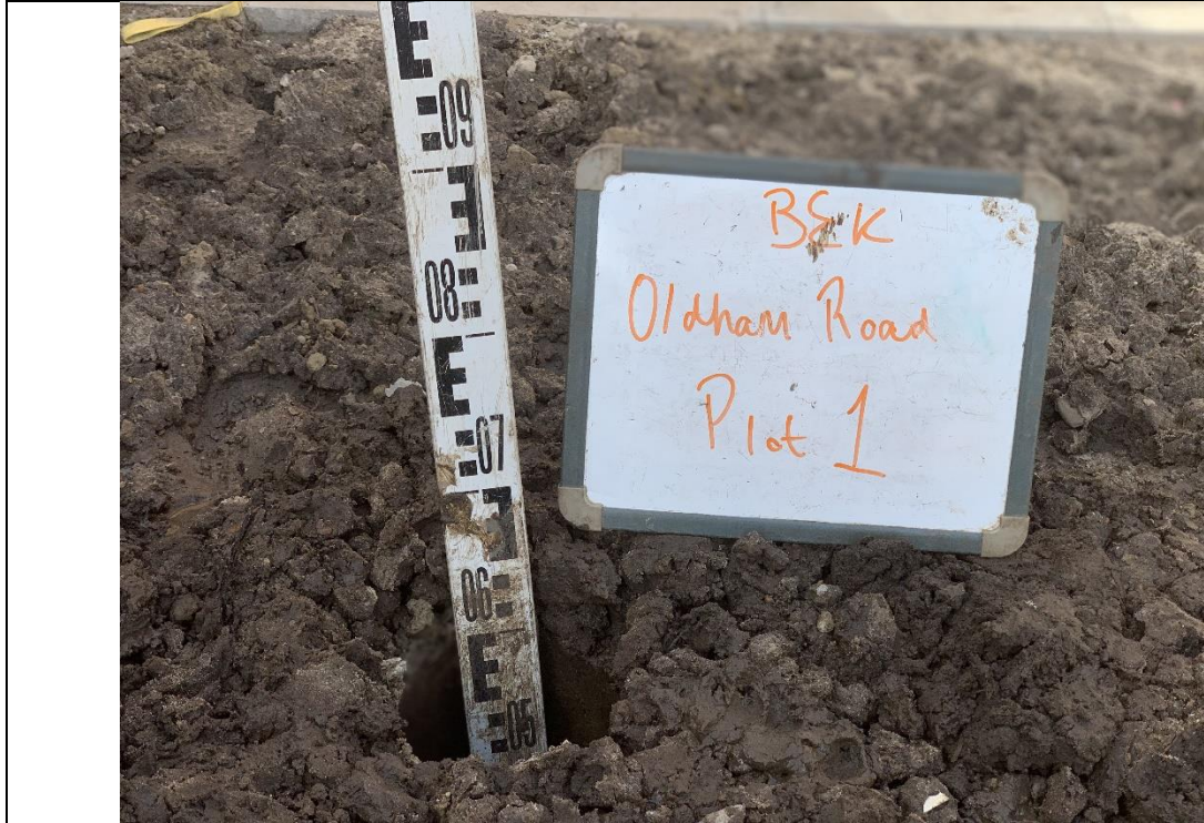
Photograph 1: Validation of Garden Capping
