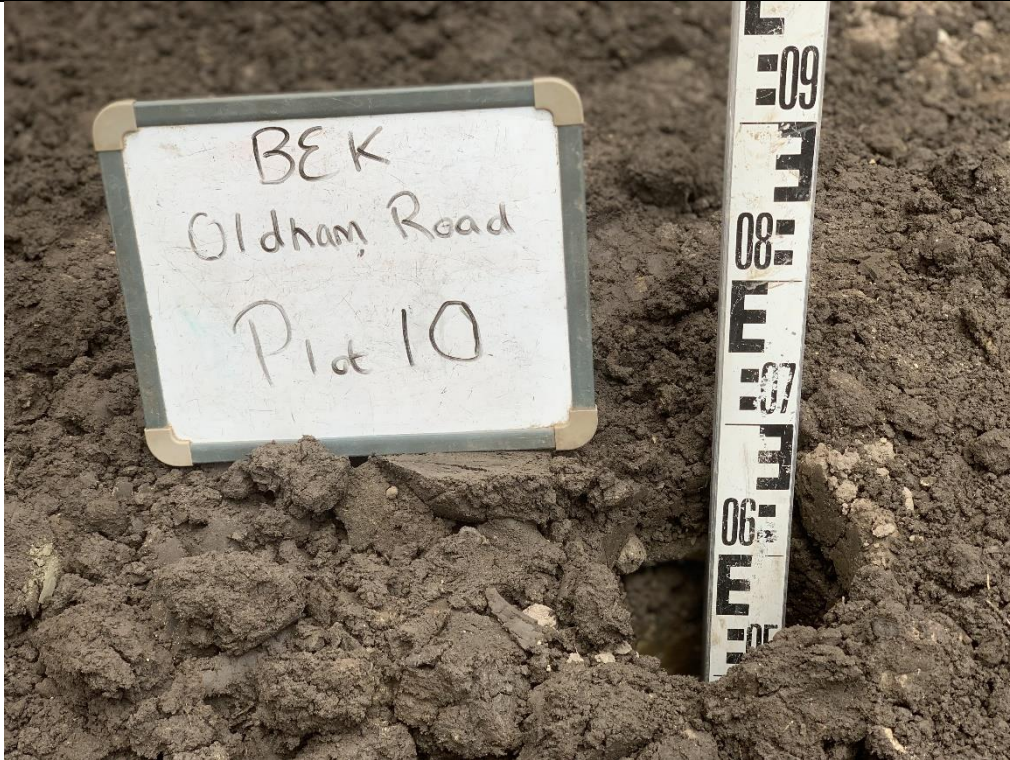
Photograph 1: Validation of Garden Capping
