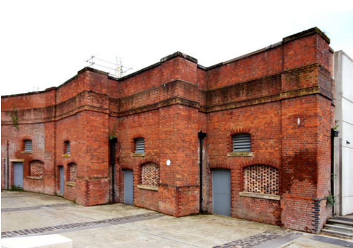
Zigzag Viaduct, Water Street
