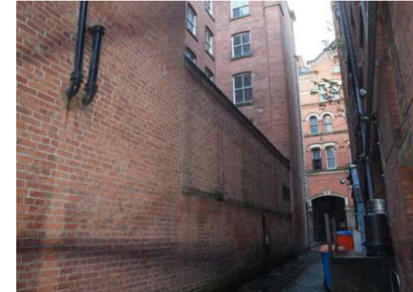
1. Alleyway wall currently demolished to be partially reconstructed with similar/reclaimed materials
