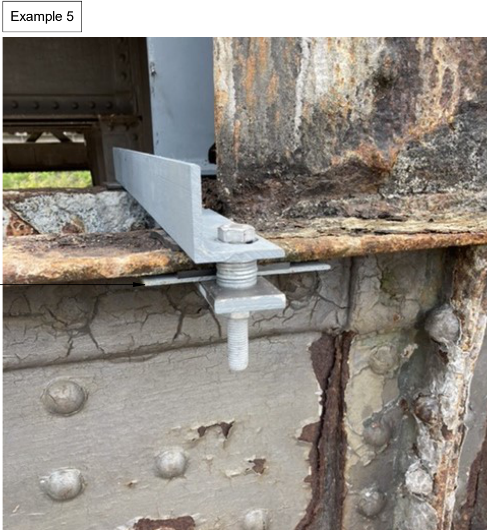
Washers as packers across top flange of bottom chord
