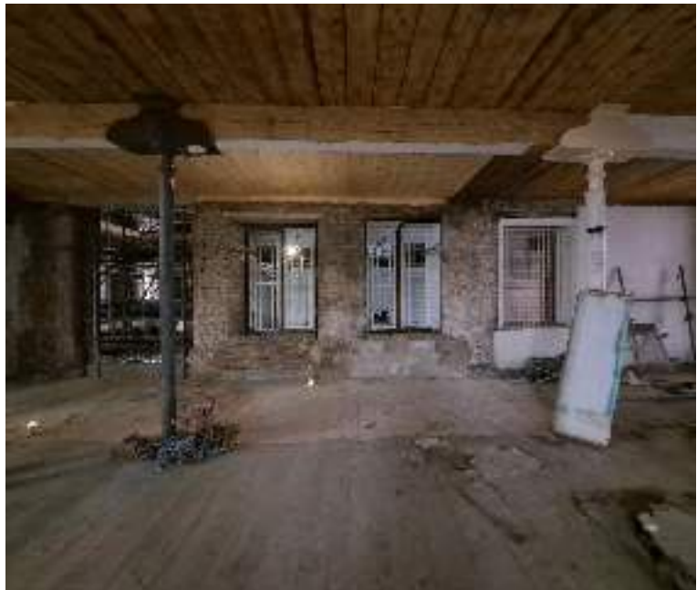
4. Column and beams to be intumescent painted
