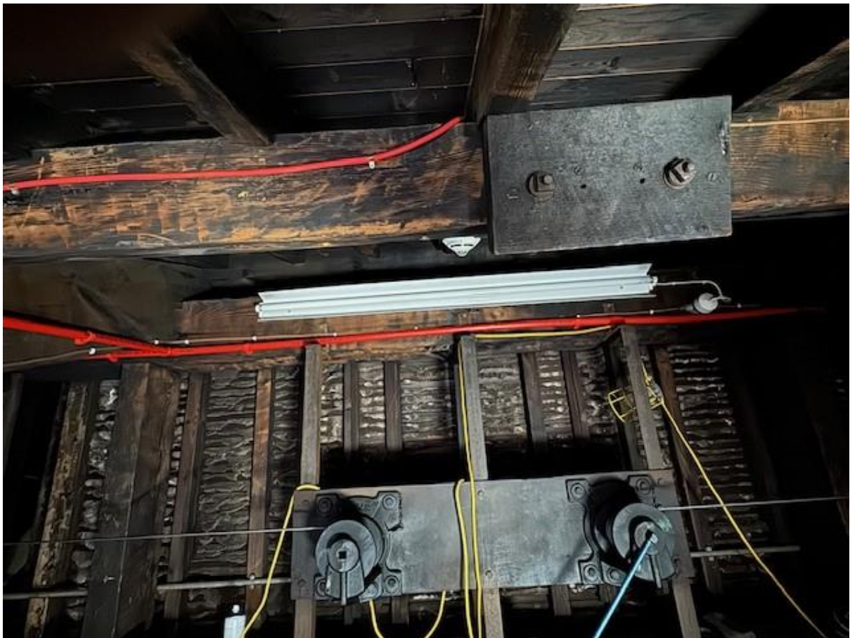
Fig 4. Internal roof space, showing timber ring beam and plaster & lathe construction. Photo by author 2024.
