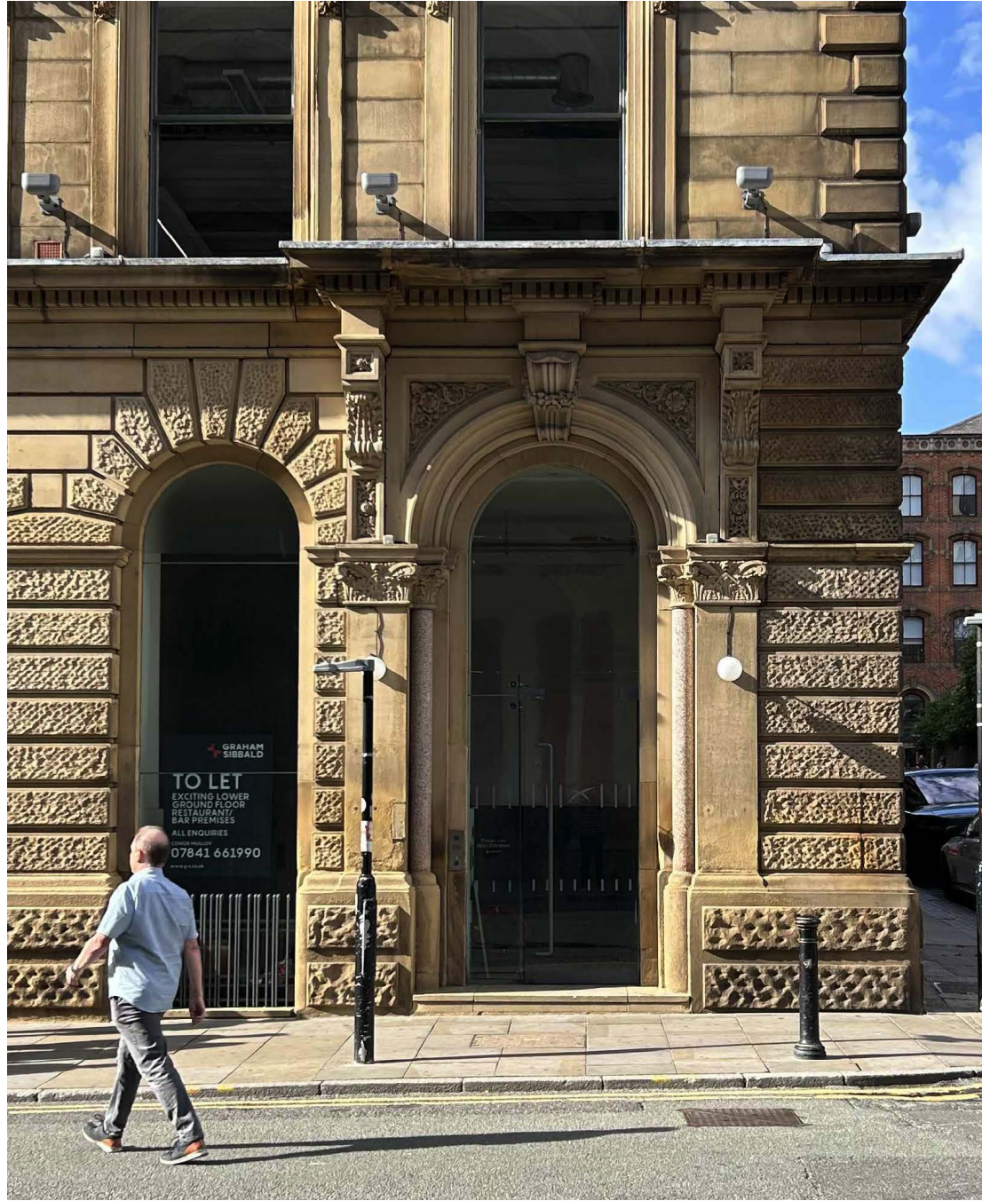
EXISTING SHOPFRONT ENTRANCE REFERENCE IMAGE
