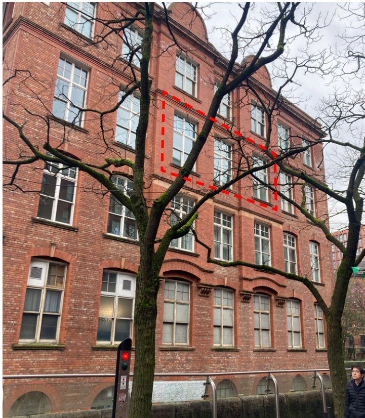
Photograph of the north elevation overlooking Canal Street with the location of the flat highlighted.
