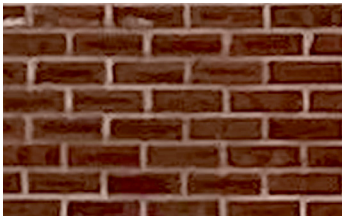
3 Example of Existing Red Brick
