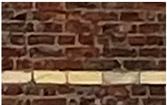
4 Example of Existing Red Brick
