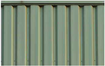
2 Profiled aluminium cladding panels
