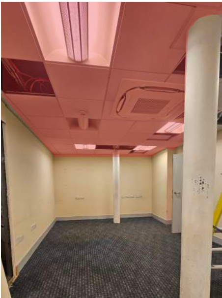
EXISTING FALSE CEILINGS TO INTEGRATE MEP TO BE DEMOLISHED.
