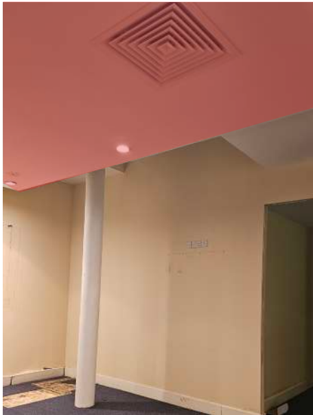
EXISTING CEILING RAFTS AND SERVICES TO BE DEMOLISHED.
