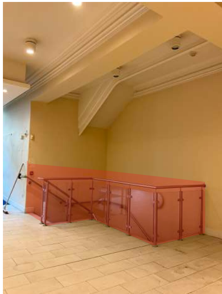
STAIRCASE TO BE DEMOLISHED, AND SLAB INFILLED
