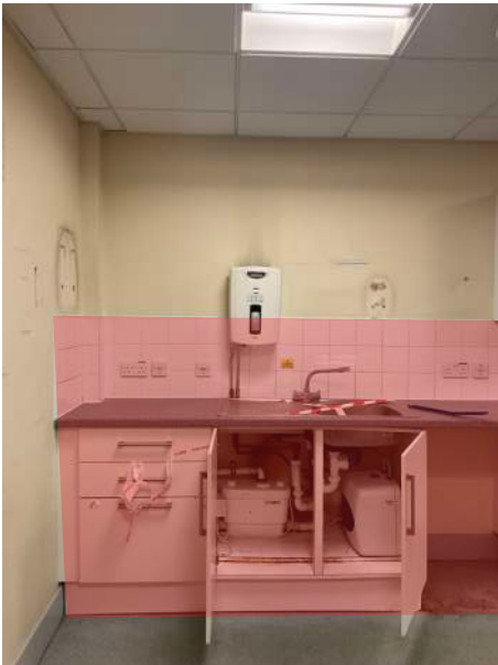
EXISTING SANITARY WARE AND MILLWORK TO BE REMOVED.
