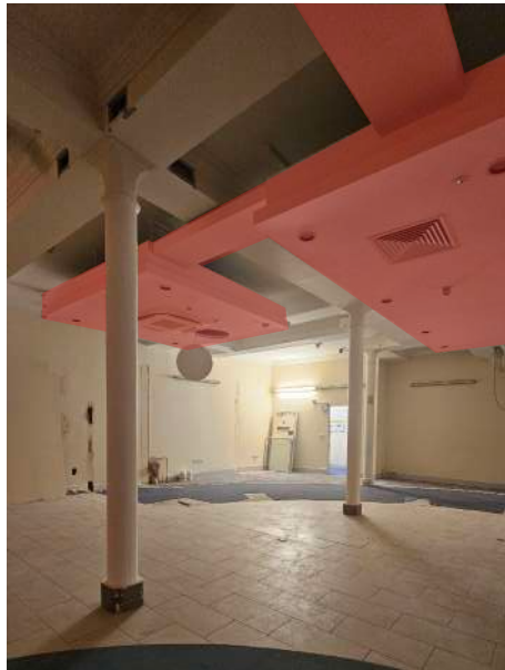
EXISTING CEILING RAFTS AND SERVICES TO BE REMOVED
