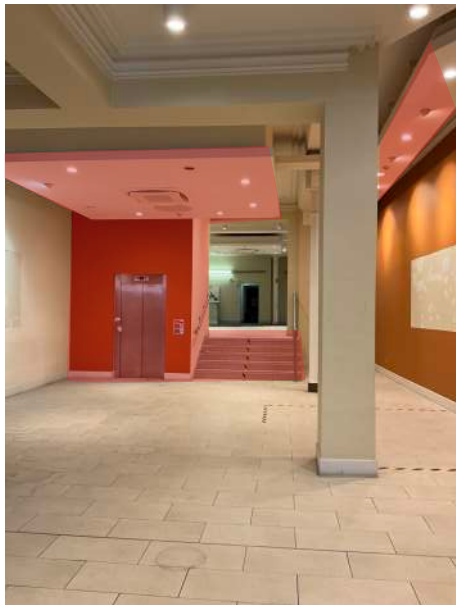
EXISTING LIFT AND STAIRCASE TO BE DEMOLISHED
