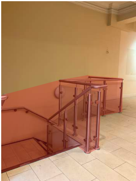
STAIRCASE TO BE DEMOLISHED, AND SLAB INFILLED
