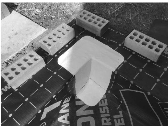
Corner detailing sealed using Juta GP SAM
