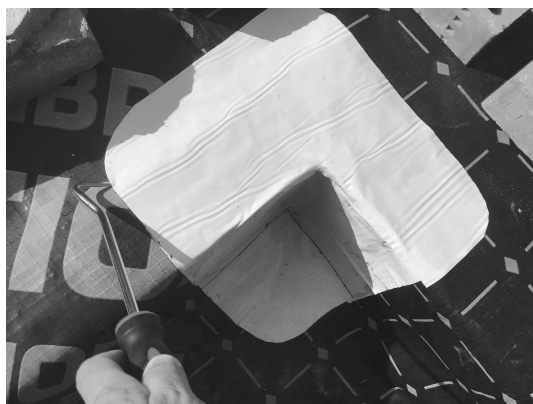
Probe test to corner detailing
