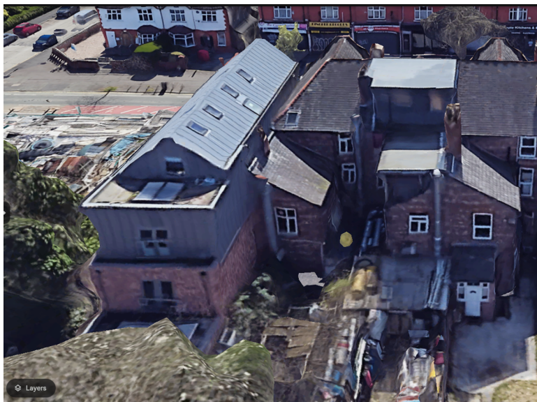
Figure 1, Rear outriggers and extensions of properties along Wilbraham Road and the applicant site.
