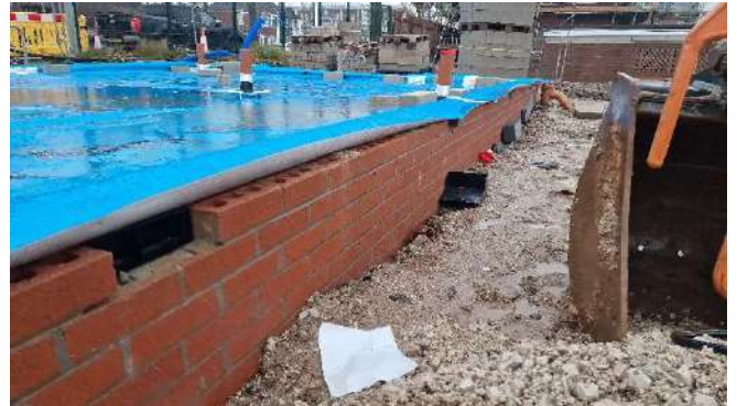
Figure 2 – Sufficient vents. Front fascia to be installed as brickwork progresses
