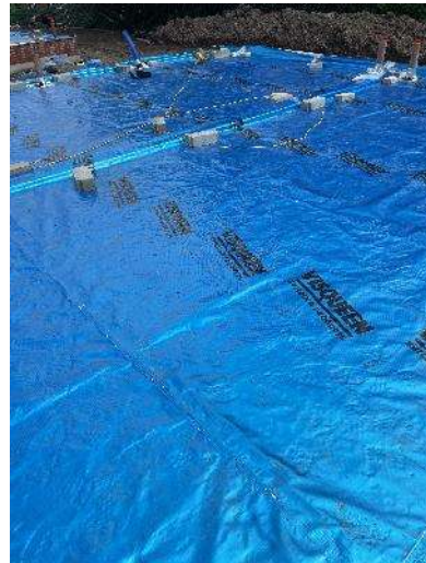
Figure 4 – Membrane in good condition.
