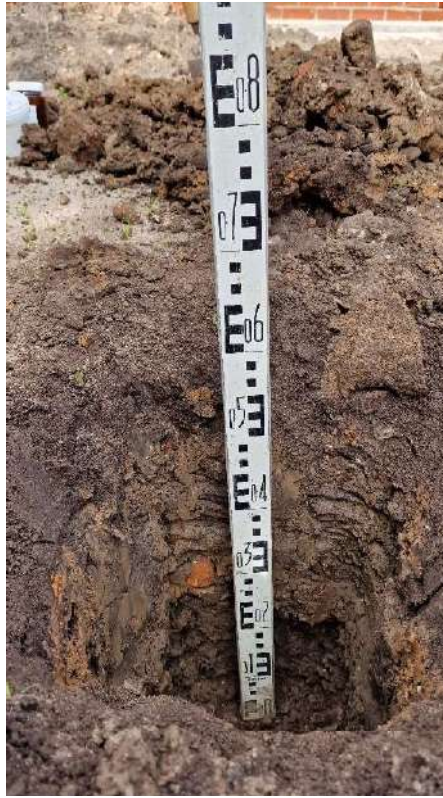
Depth of pit demonstrated at 600mm
