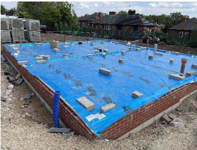
Figure 1 – General view of the plot. Sufficient coverage of cavities.
