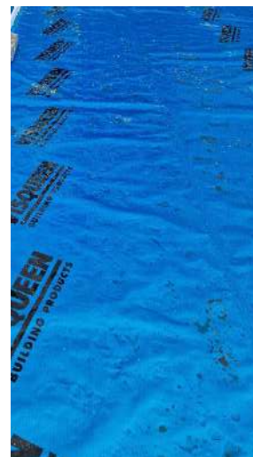
Figure 6 – Joints are correctly hand welded.
