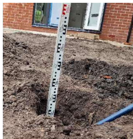
Depth of pit demonstrated at 600mm
