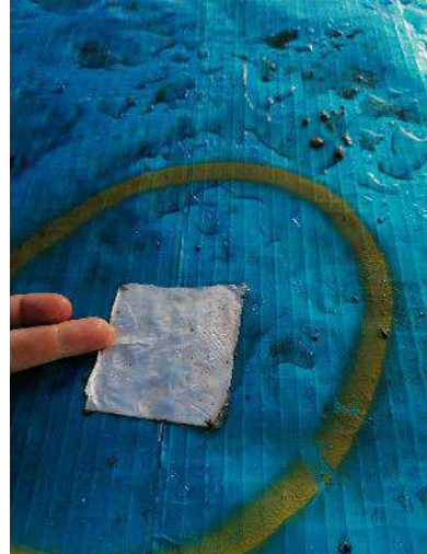
Figure 4 – Gaps in welding have been correctly patched.
