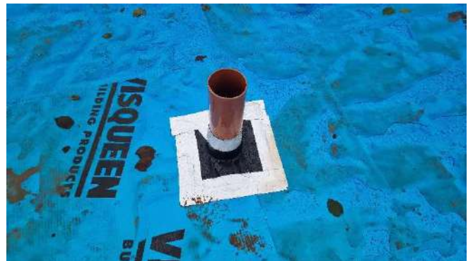
Figure 6 – Service entries sealed and secure.
