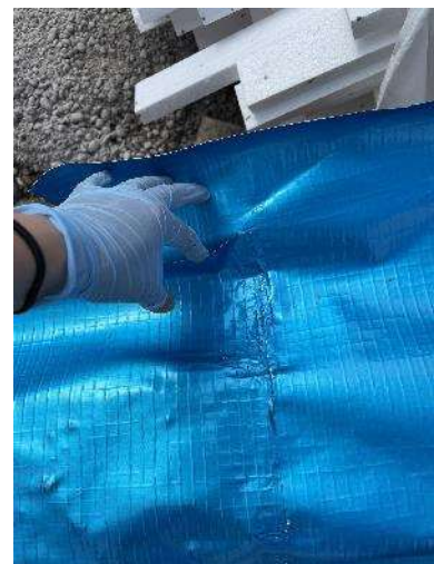
Figure 6 – Joints are hand welded.
