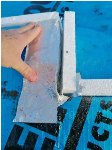
Figure 3 – Gaps in corners correctly patched.
