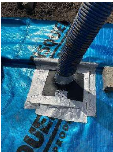
Figure 5 – Service entries sealed on return visit.
