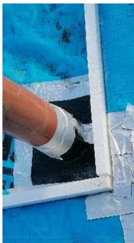
Figure 5 – Gaps in service entry bases correctly sealed.
