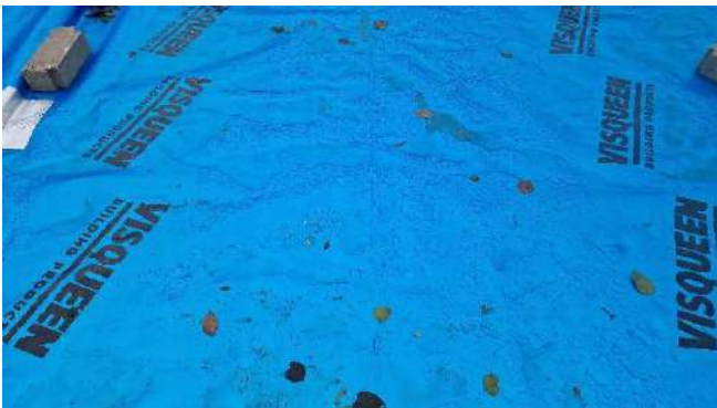
Figure 5 – Hand Welded Seams
