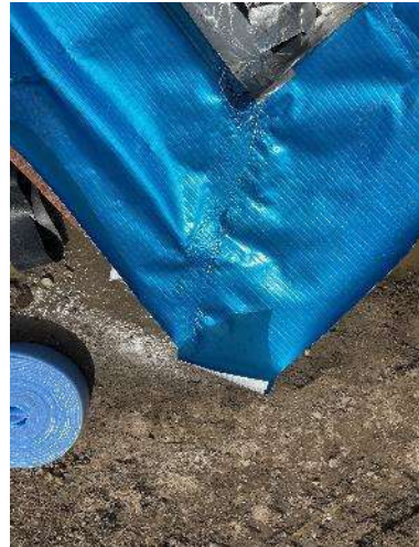
Figure 6 – Joints and corners are hand welded.
