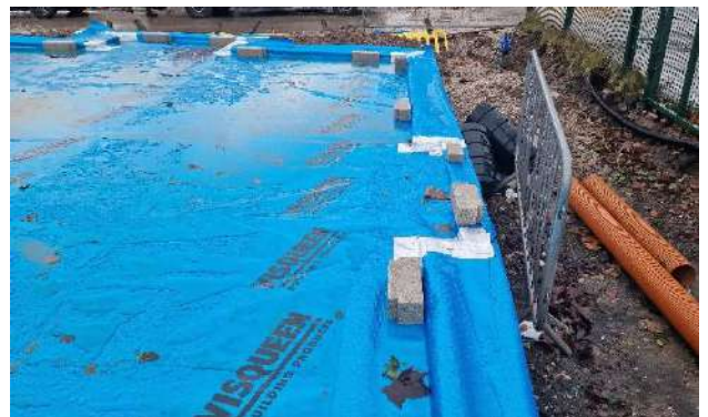
Figure 4 – Sufficient cavity cover.
