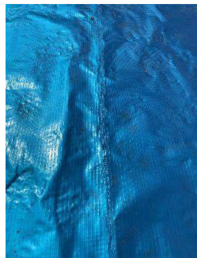
Figure 6 – Joints are hand welded.
