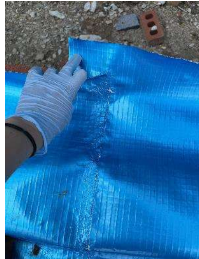
Figure 6 – Joints are correctly hand welded.
