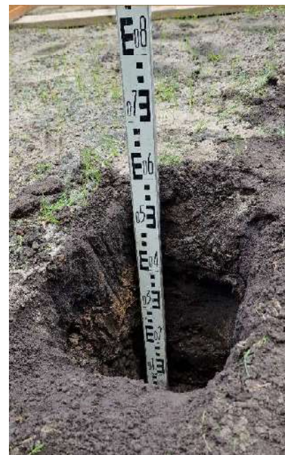
Depth of pit demonstrated at 600mm
