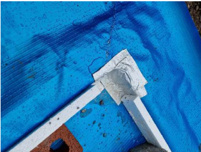
Figure 3 – Corners installed correctly using hand welding and detailing tape.
