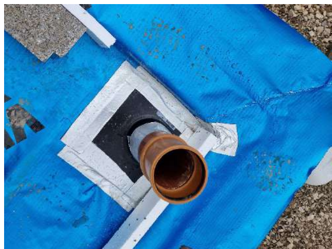
Figure 5 – Service entries sealed and secure.
