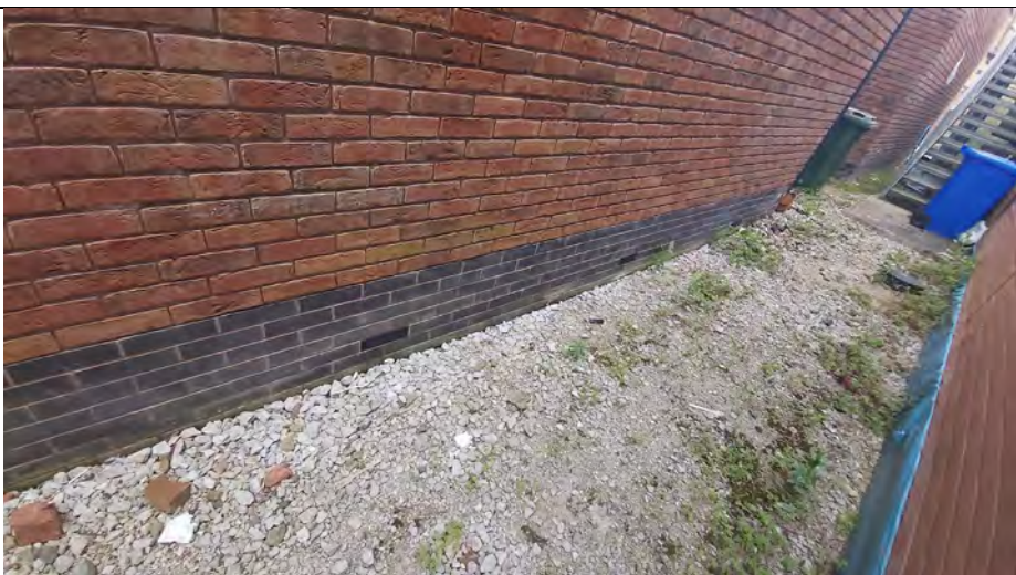
14. Airbricks 23, 24, and 25 obscured by foliage.
