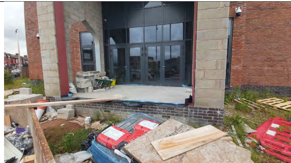
1. Front entrance to the mosque on the NW side, looking SE. Vents 1, 2, 3 visible at least 5 bricks from the ground (350mm).
