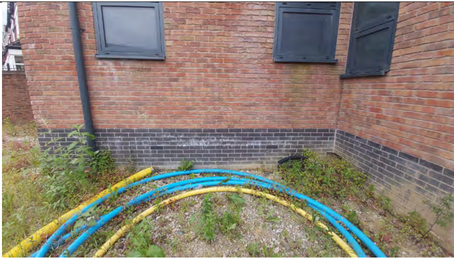
3. External airbricks 5 and 6, at 400mm height from ground level.
