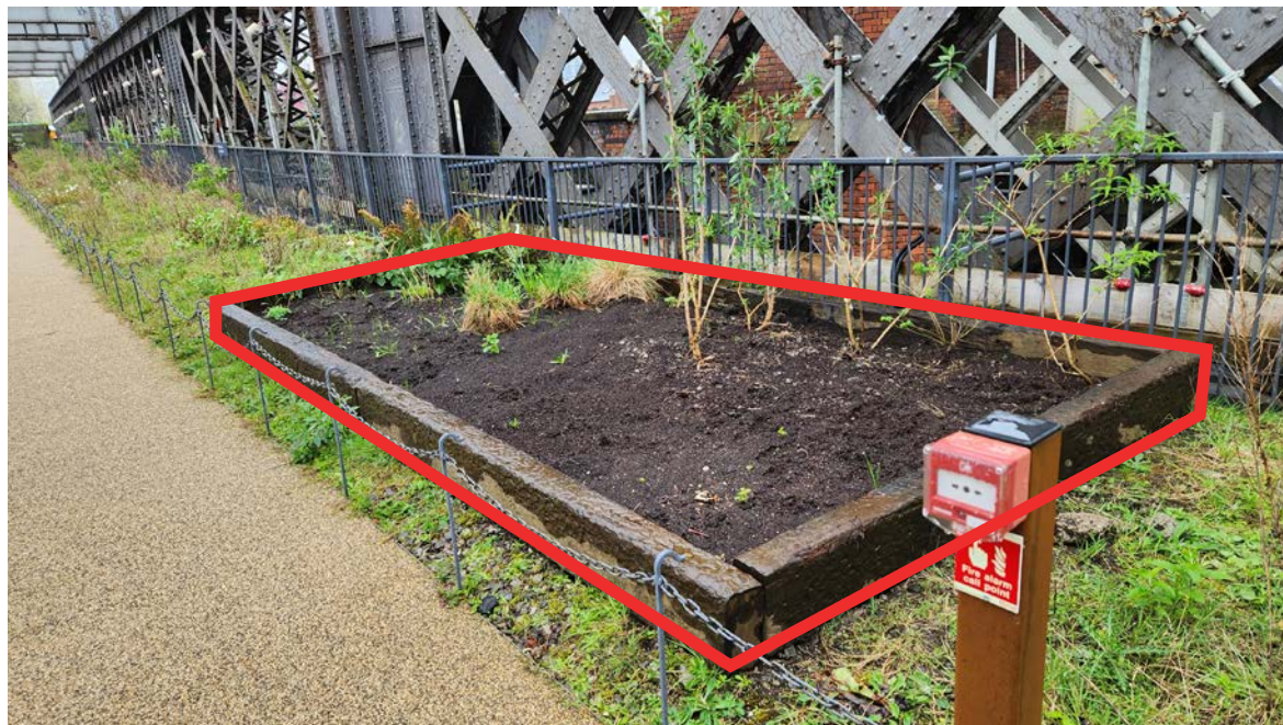
Timber sleeper planting bed in Phase 01
