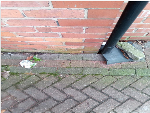
Fig 1.1: Trial Hole 1 Location
