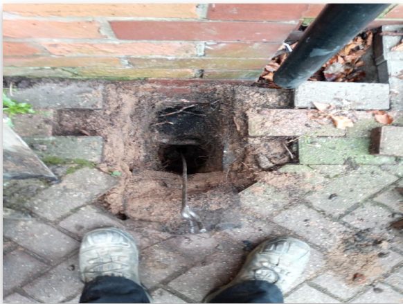
Fig 1.2: Trial Hole 1 Footing
