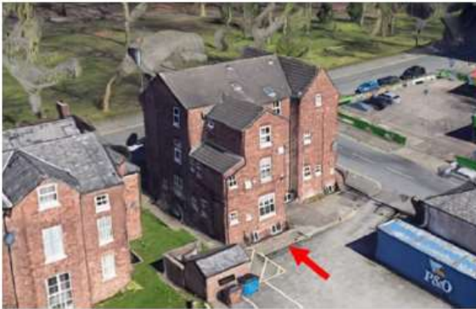
Demolition Start Point
