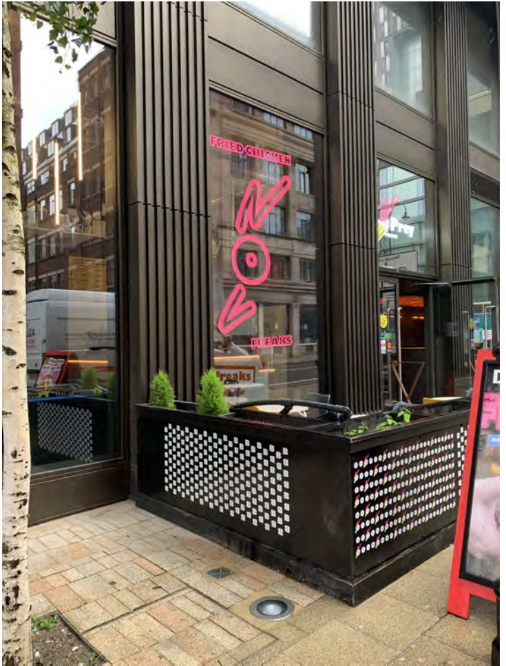
Existing signage example
