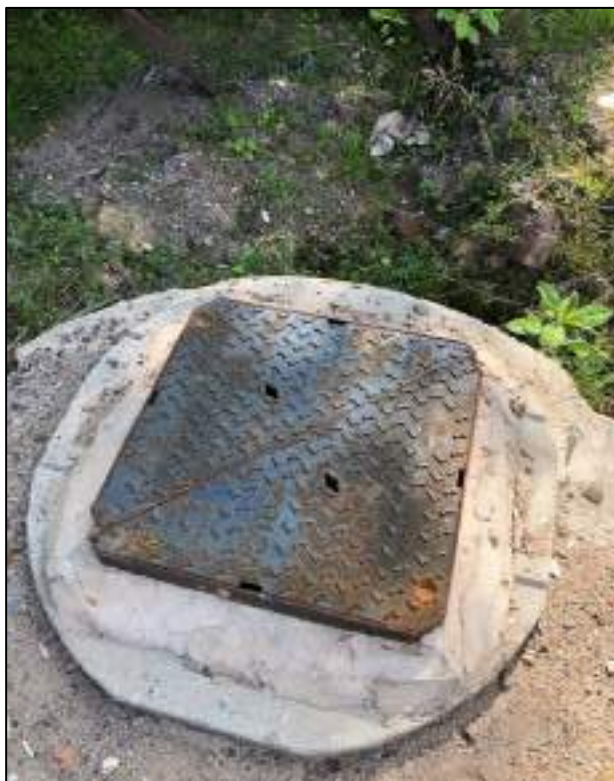
Drain cover in southeast corner of site
