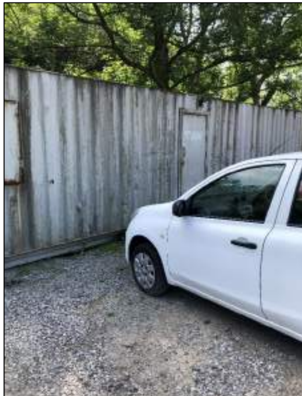
Steel shed on southern boundary
