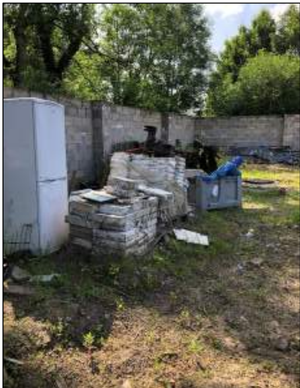
Material left on site
