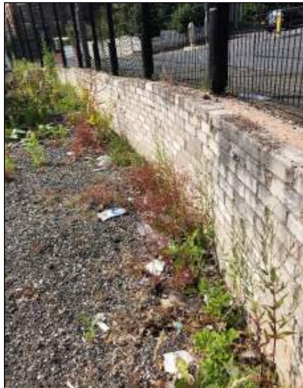
Retaining wall along northeast boundary
