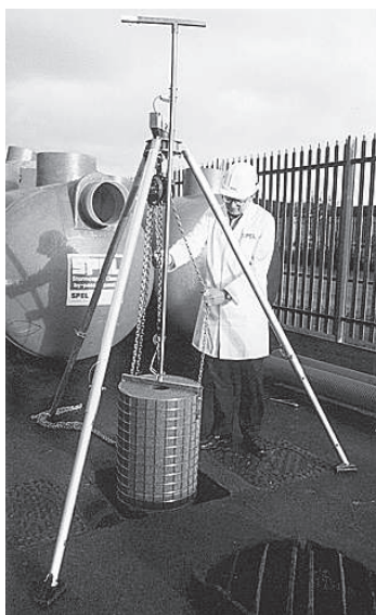
Step 8 – As the coalescer unit rises, steer the lifting handle past the tripod head and hoist to allow continued lifting of the coalescer unit.
