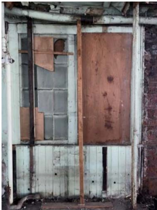
Existing Hoist timber doors
