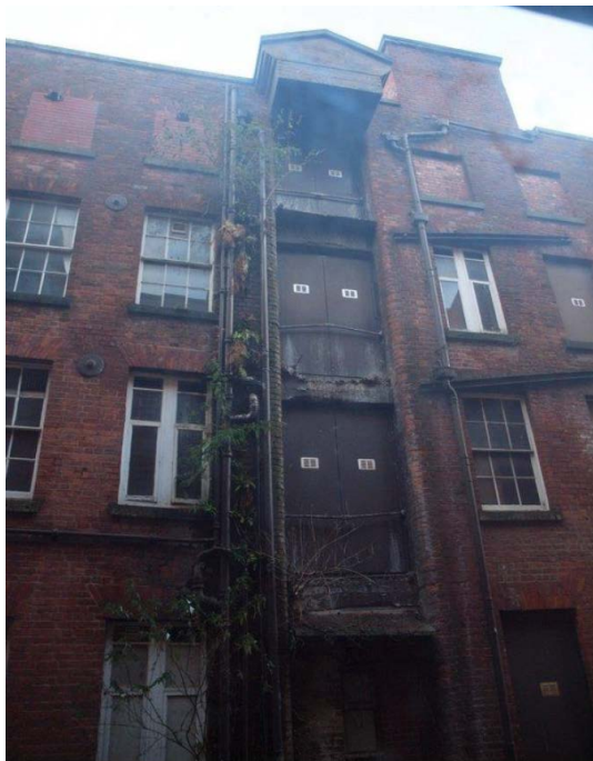
Potografic record prior to strip-out works
