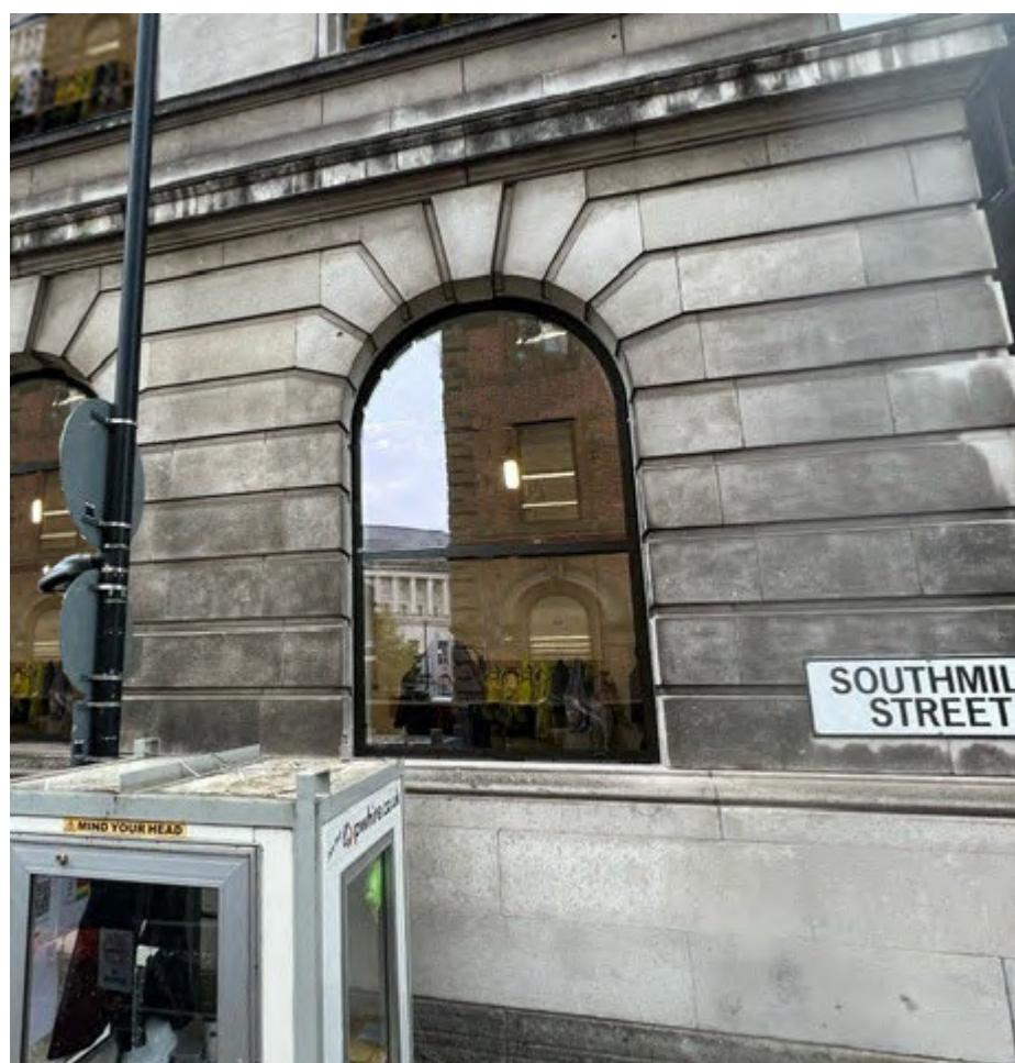
Lowered transom (low) Vertical and splayed metal members removed
