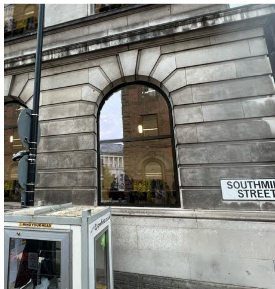
Lowered transom (mid) Vertical and splayed metal members removed
