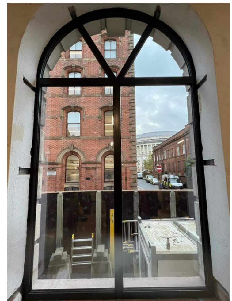
RIBA Stage 4/5 drawings - Current condition Southmill Building Windows
