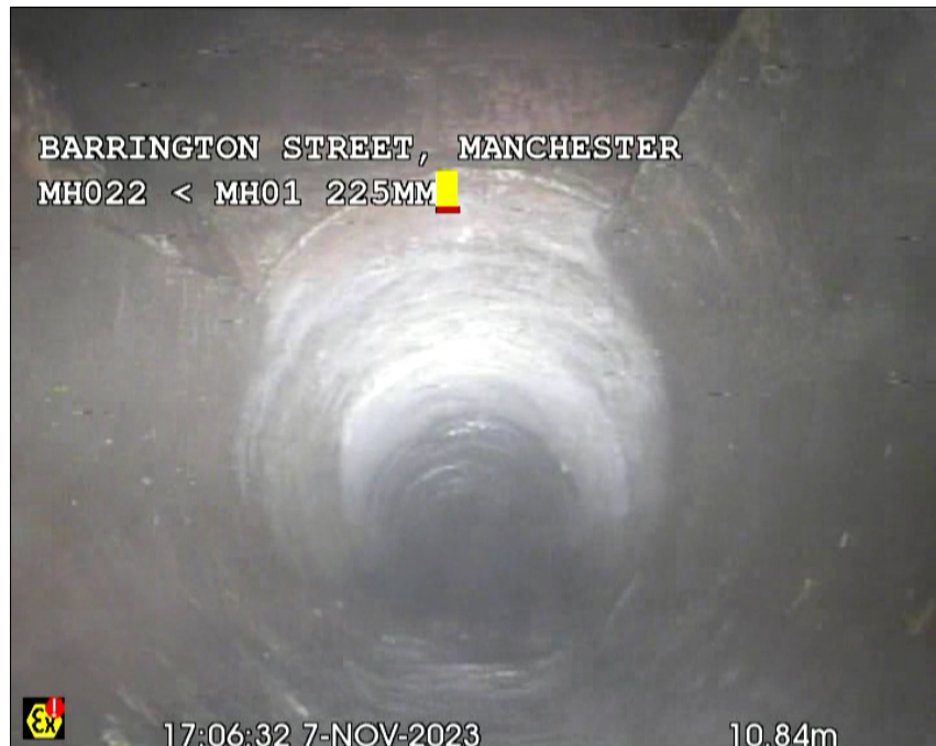
Photo: 1_1_4_A.jpg 10.84m, Finish node type, manhole reference number: MH01
