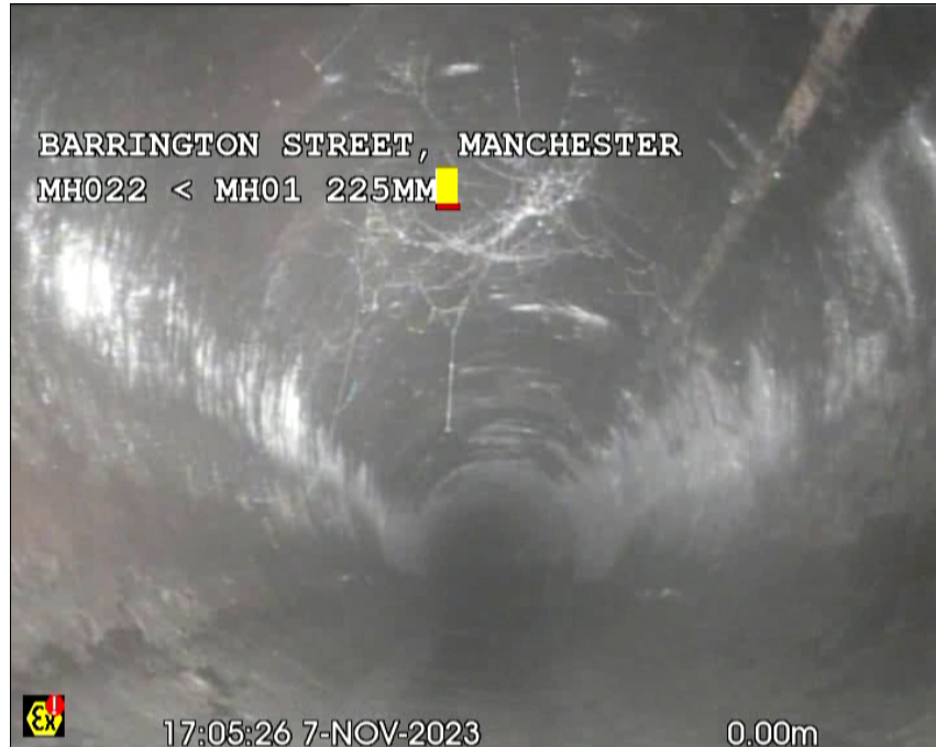
Photo: 1_1_1_A.jpg 0m, Start node type, manhole, reference number : MH022
