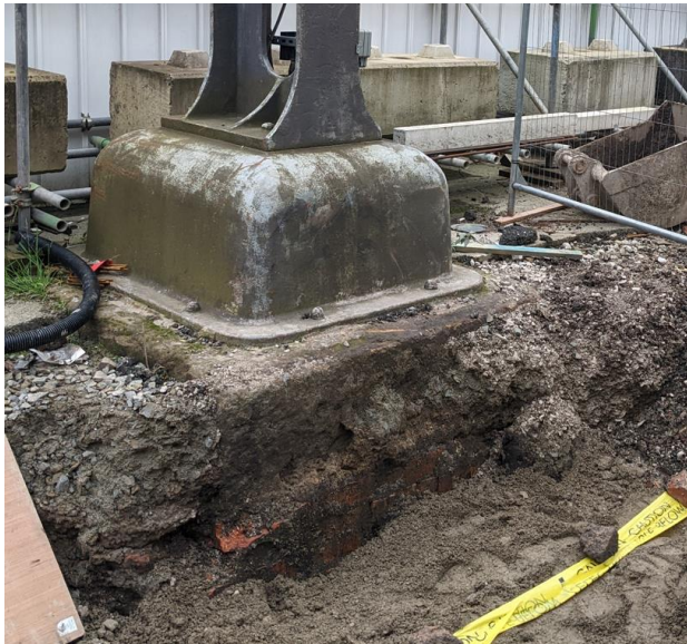
Figure 2-9 Plinth / foundation detail
