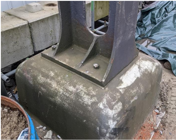
Figure 2-10 Plinth detail
