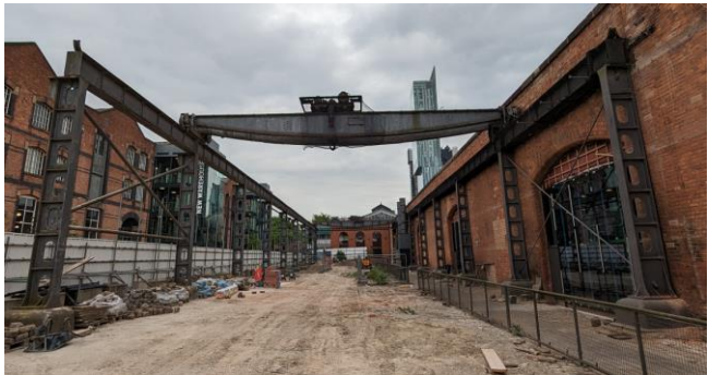
Figure 2-14 General view from west
