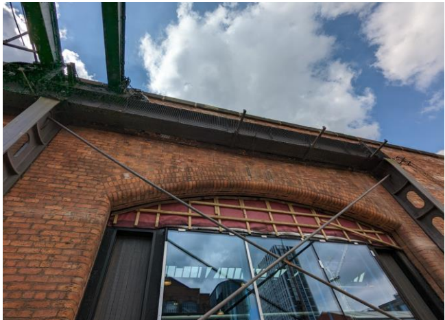
Figure 2-17 South cross bracing
