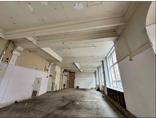
Existing Sprinkler Installation
