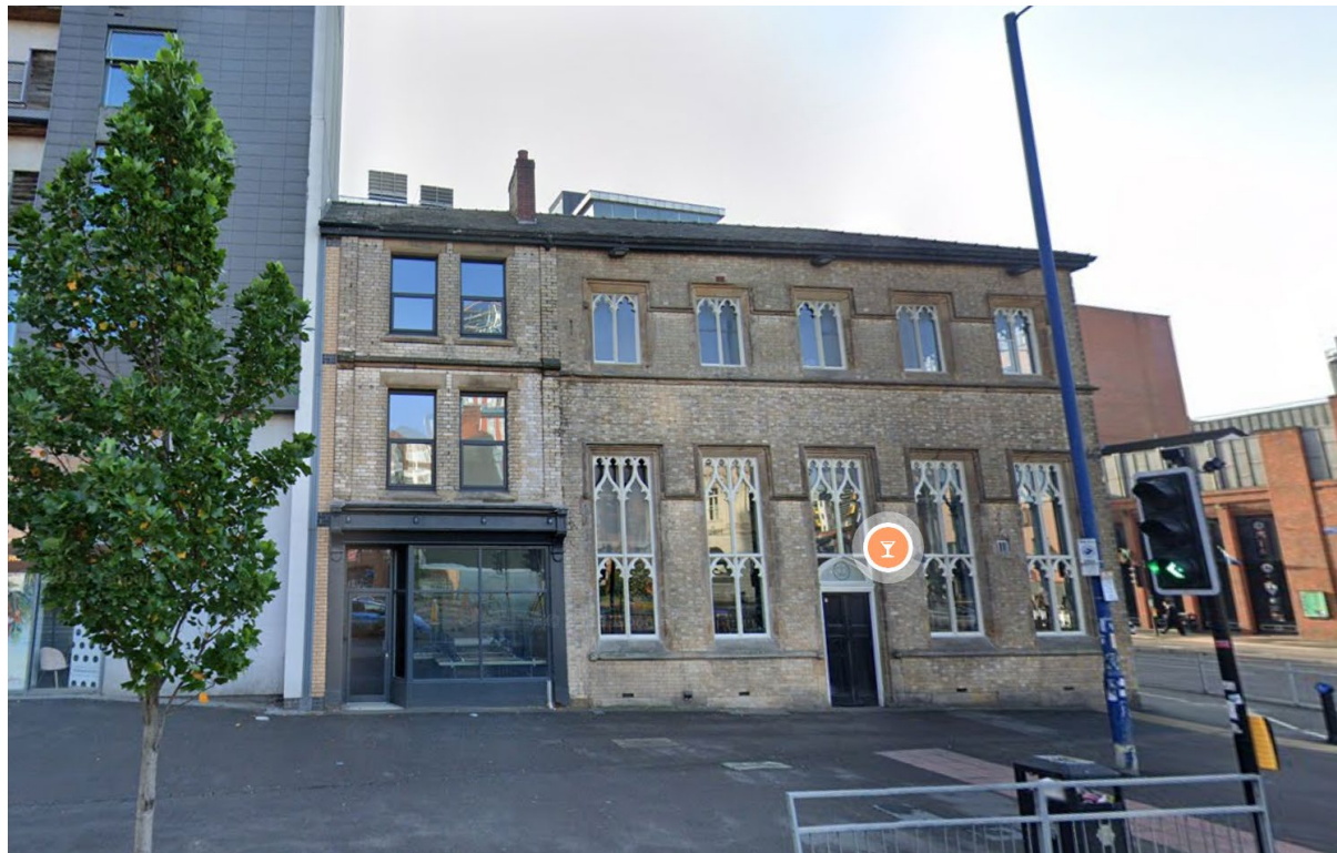
^ Figure 2: Site's Oldham Road frontage (taken from Google Maps)
