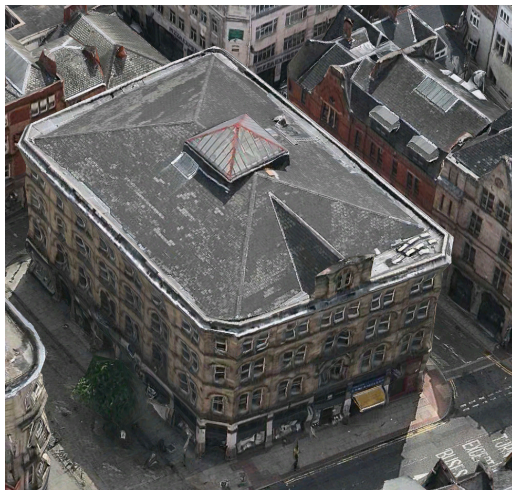
Image 2: Aerial image of the property showing the altered roof with central pyramid roof light.
