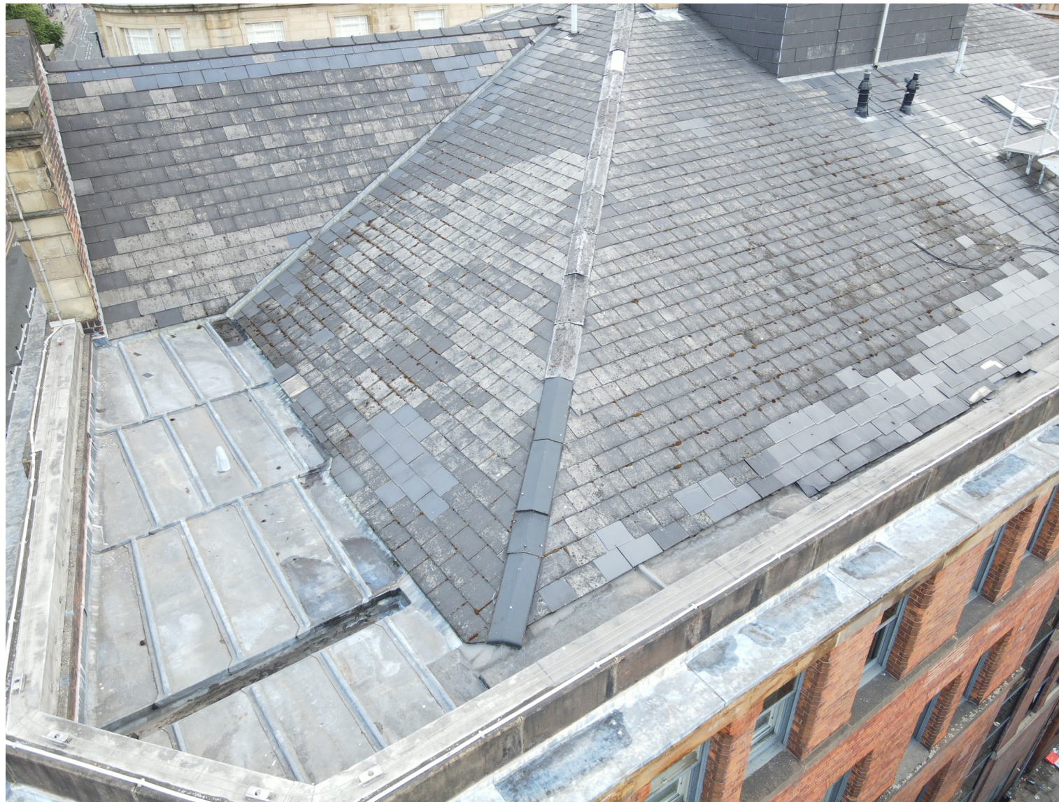
Image 21: Contemporary aerial view of roof showing composite tiles and lead.
