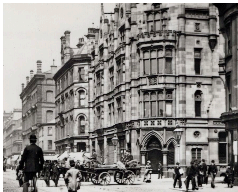
Image 6: Historic photograph of building, as viewed from Deansgate in late 19th century.
