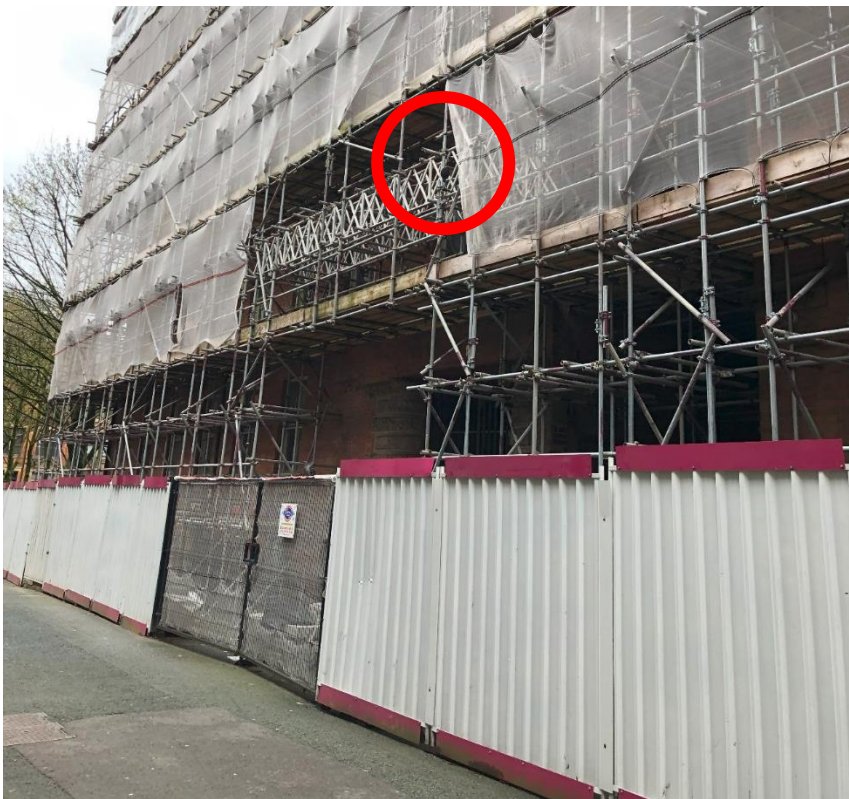
Figure 3 Unattended measurement position overlooking Richmond Street
