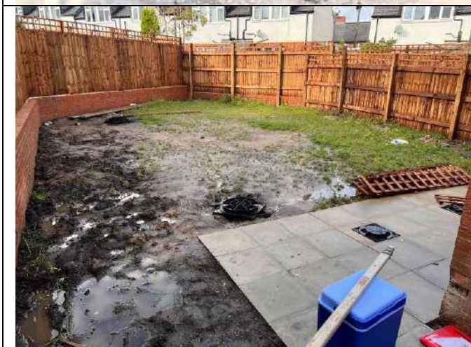
Photograph 16: View showing rear garden (Plot 11).
