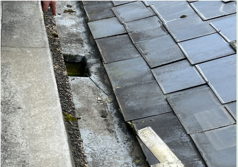
DETAIL OF GUTTER AND OUTLET
