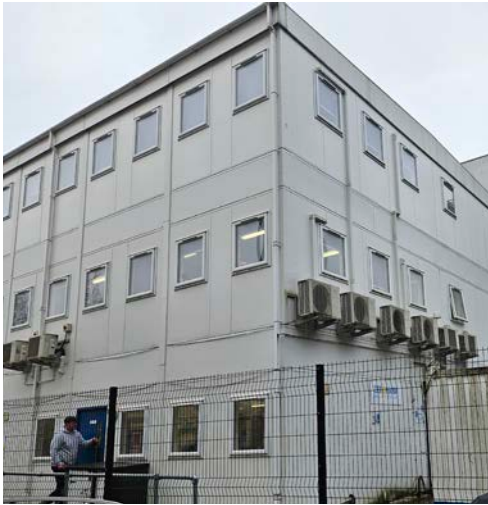
Existing Cabin's Exterior
