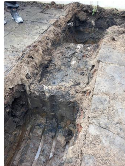
Photo No.4: Second angle of obstruction showing corrugated imprint on concrete to either side of feature and clay infill
