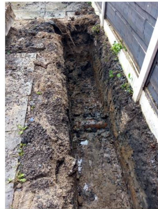
Photo No.2: Facing east showing the same footing section
