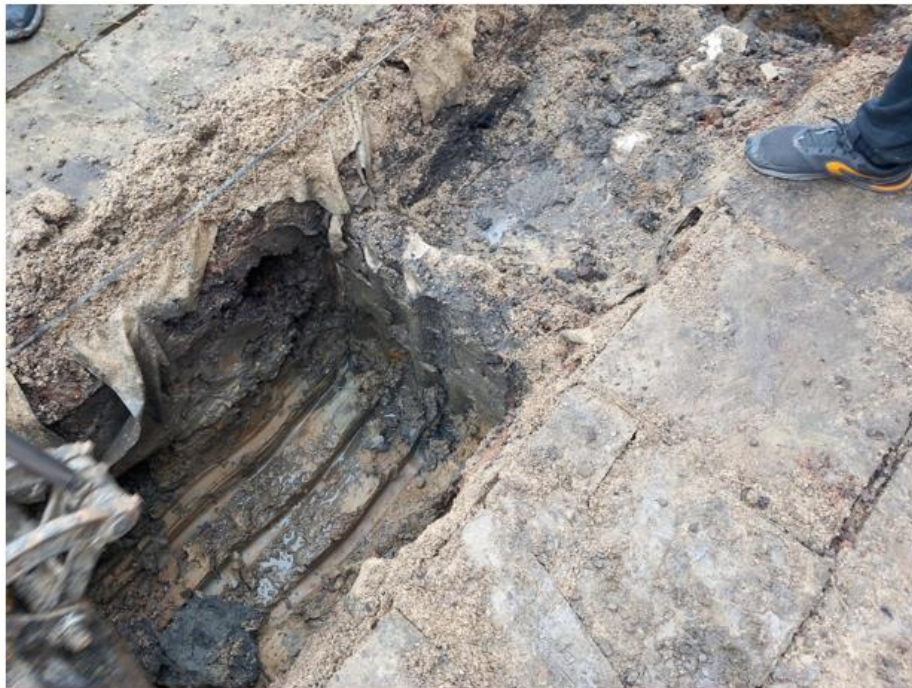
Photo No.3: Concrete obstruction (possible former Anderson Shelter) in southern extent of north-south footing section
