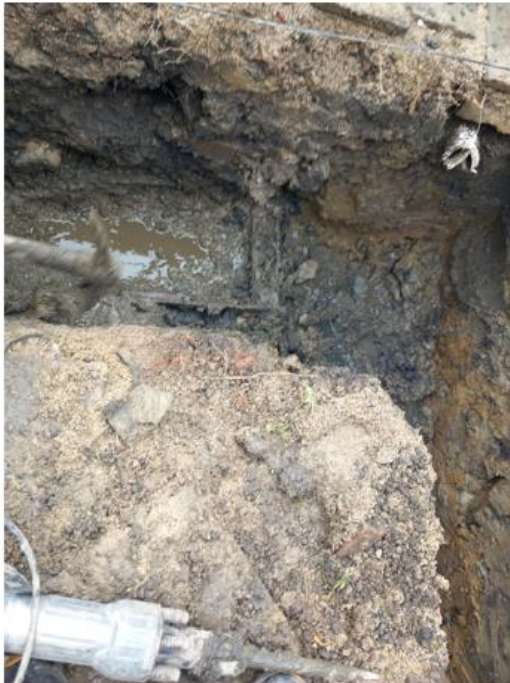
Photo No.7: Concrete obstruction removed exposing the former metal structuring / base to likely corrugated tin
