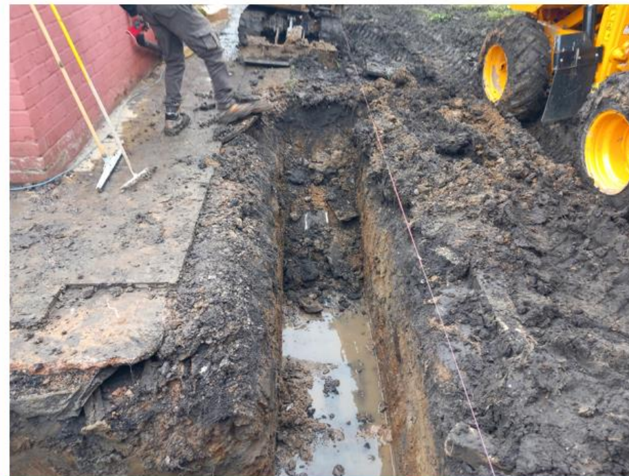
Photo No.10: Facing west from the NE extent of the footings
