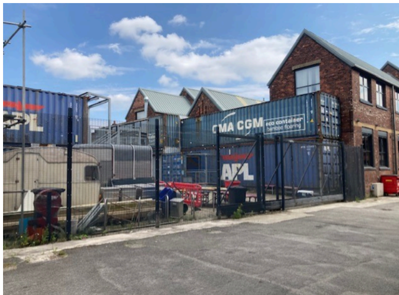
View of building rear
