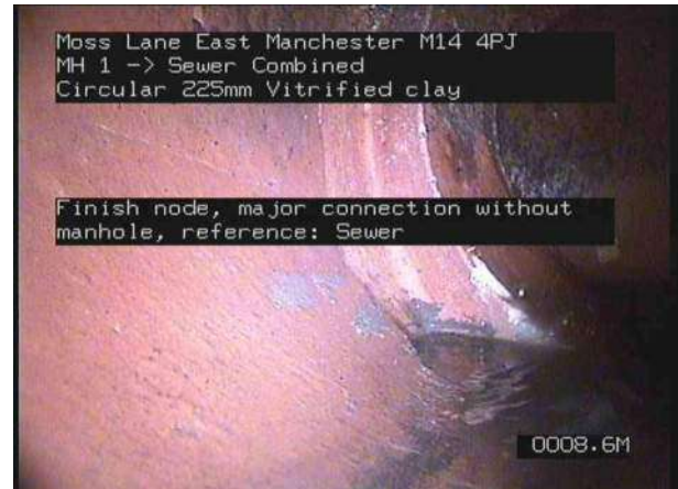
MH 1X_2d7e1770-ffde-4613-a7cd-1d9af16ecad4_20220722_1349 01_153.jpg, 00:01:21, 8.60 m Finish node, major connection without manhole, reference: Sewer
