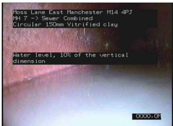
MH 7X_ee1045f8-42b1-481c-af9b-031247f28254_20220722_1036 26_994.jpg, 00:00:15, 0.00 m Water level, 10% of the vertical dimension
