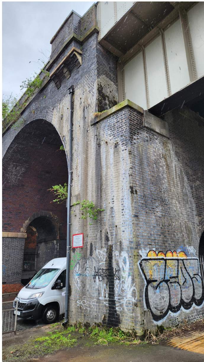
Existing condition of Arch 272 Pier
