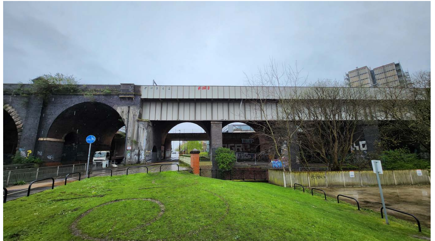
View toward masonry viaduct from Porcelanosa land
