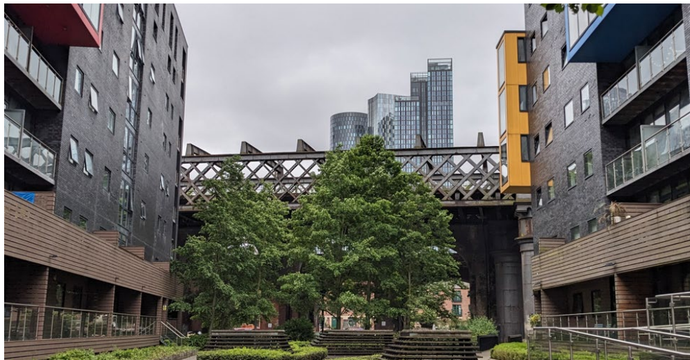
Figure 4 - View of Castlefield Viaduct from Potato Wharf (June 2024)
