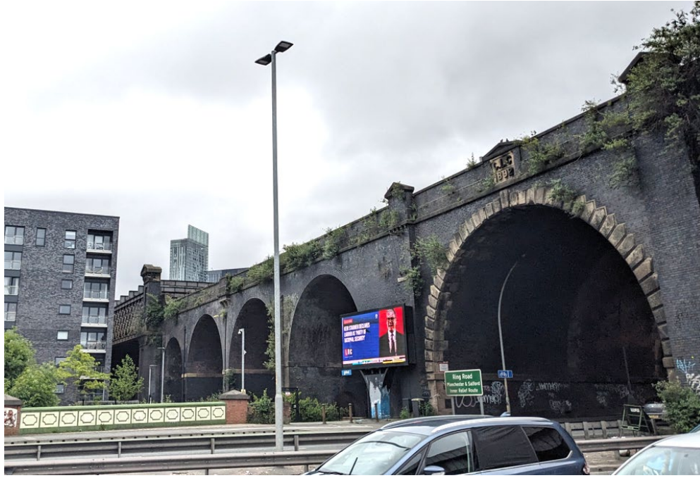
Figure 8 - View of the non-listed segment of the viaduct from Egerton Street (June 2024)
