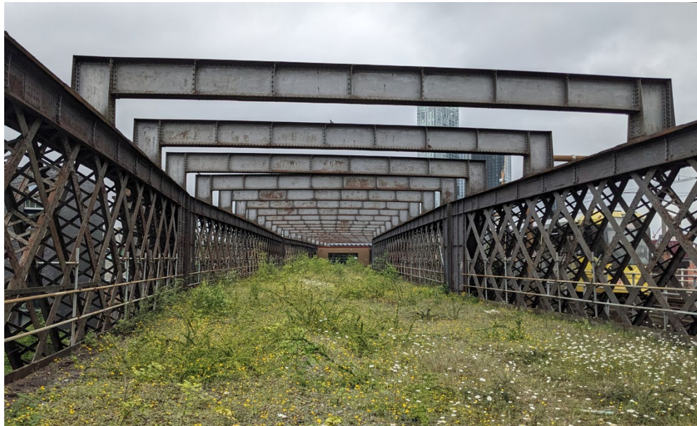
Figure 7 - Phase 2, facing north-east. The existing Engagement Centre is visible in the background, as is a passing Metrolink tram to the south (June 2024)
