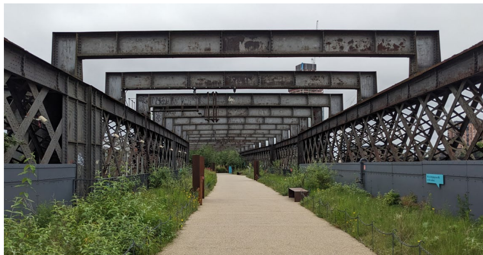
Figure 6 – Phase 1 main walkway, showing lattice girders and overhead bracing (June 2024)
