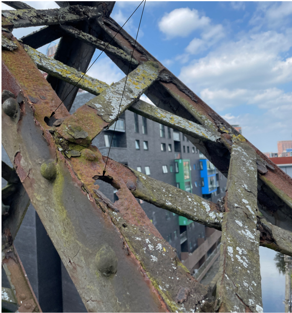
Example 3 - loss of section to inner angle, either side of X-bracing connection - at least 2 holes per length of outstand
